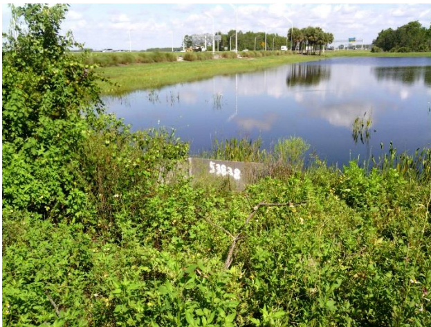
Figure 10 Overgrown structure in pond east of SR 528.
