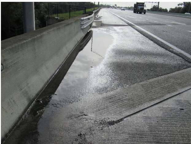
Figure 7 Ponding water on SR 414 Bridge over CR 435.
