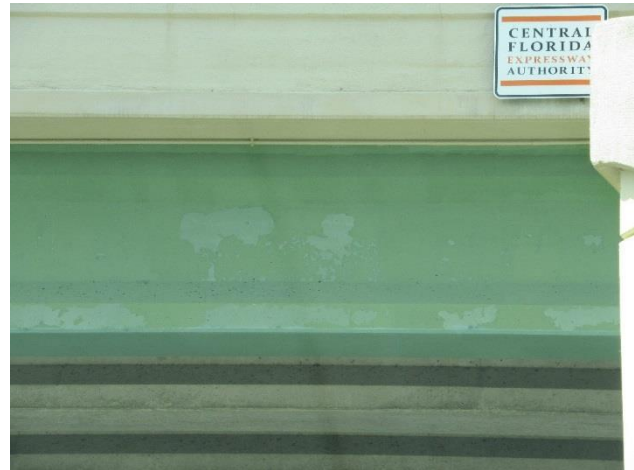
Figure 11 Peeling beam coating Lee Vista Boulevard.
