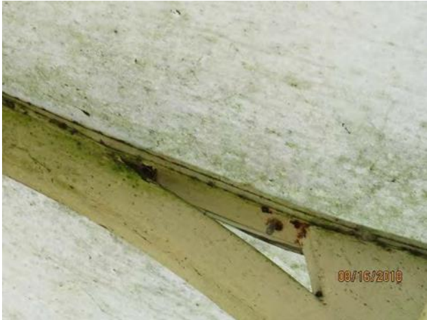
Figure 19 Mold and mildew on canopy of Dallas Mainline Plaza pedestrian bridge.
