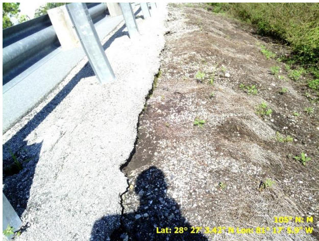
Figure 17 Roadside erosion adjacent to SR 528 east of Beachline Main.
