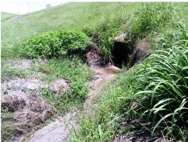
Figure 13 Drainage structure erosion southbound SR 429 at Franklin Street
