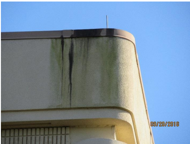
Figure 15 Mold growing on parapet of SR 429 New Independence Plaza.
