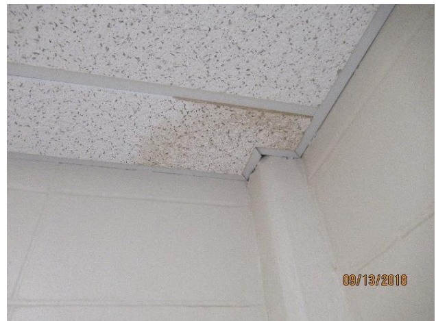
Figure 9 Damaged ceiling tile Coral Hills Mainline IT room.
