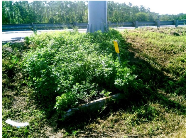
Figure 16 Overgrown drainage structure south of Johns Road.
