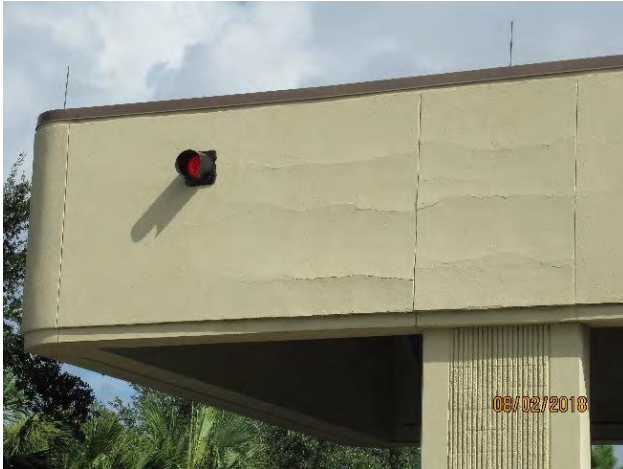
Figure 12 Building façade damage SR 417 Lee Vista on ramp (isolated occurrence).
