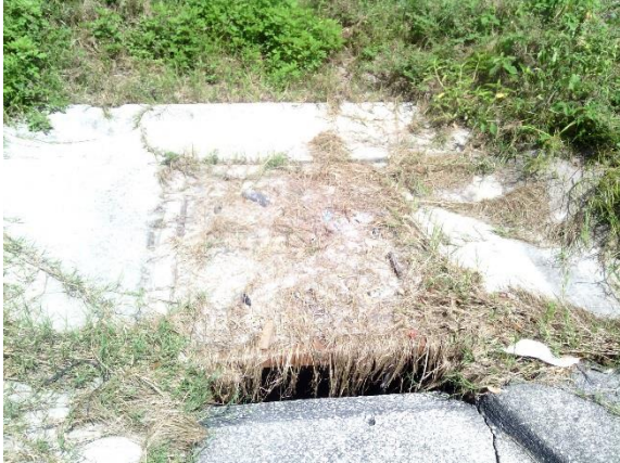
Figure 6 Obstructed drainage / flume structure at SR 414 south of Lakeville Road.
