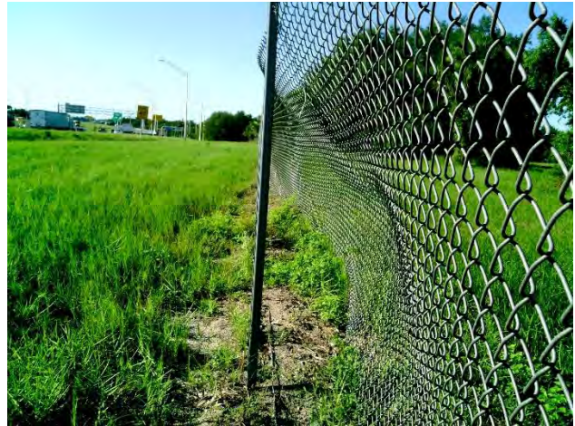
Figure 14: SR 429 fence fabric missing ties.
