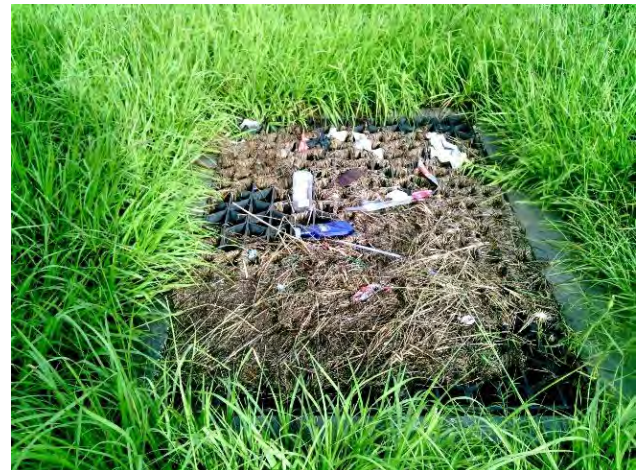
Figure 6: Obstructed drainage structure at SR 414 east of Ocoee Apopka Road.
