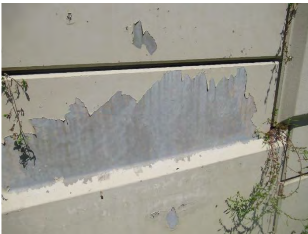
Figure 11: SR 417 over SR 50 MSE wall coating failing.
