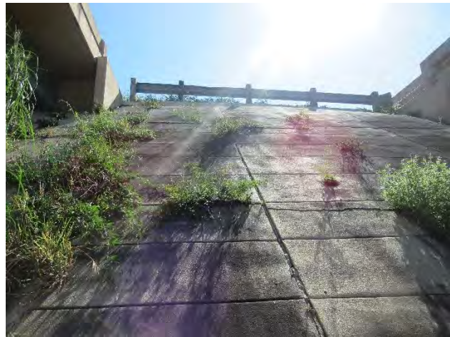
Figure 18: SR 528 over Dallas Boulevard overgrown slope pavement.
