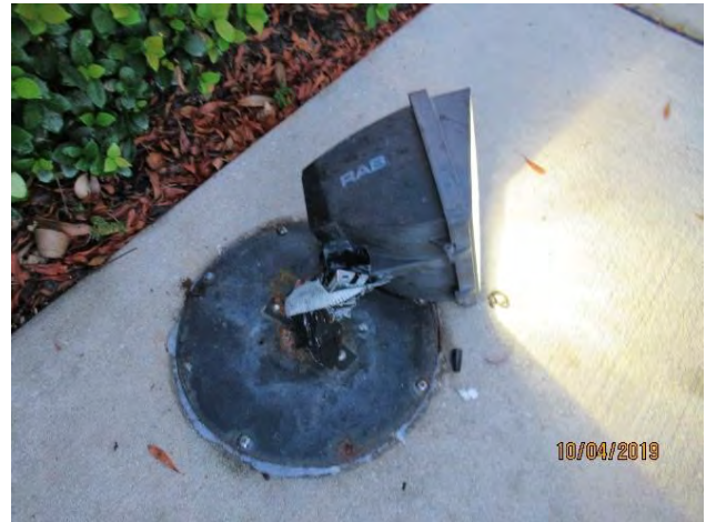
Figure 9: Broken flag pole luminaire at Coral Hills Mainline Plaza.
