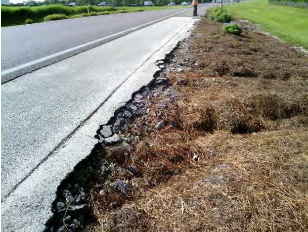
Figure 10: SR 417 Erosion along lane edge (Lee Vista Boulevard Southbound on Ramp).
