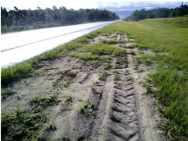
Figure 20: SR 538 (Poinciana Parkway) minor roadside erosion.
