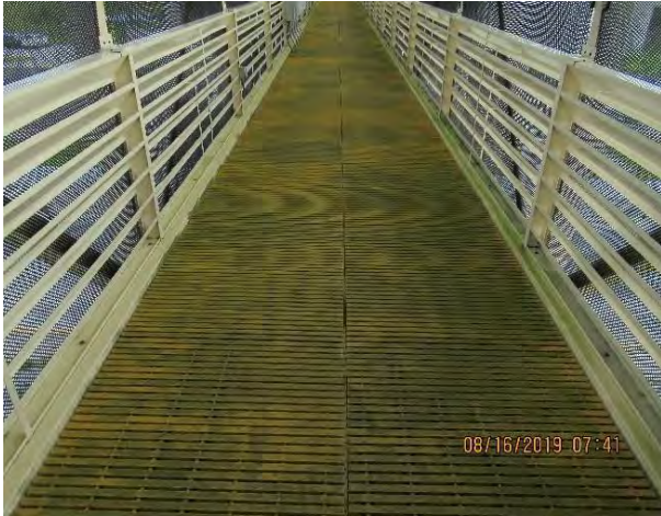
Figure 19: Dallas Mainline Pedestrian Bridge minor mold growth.
