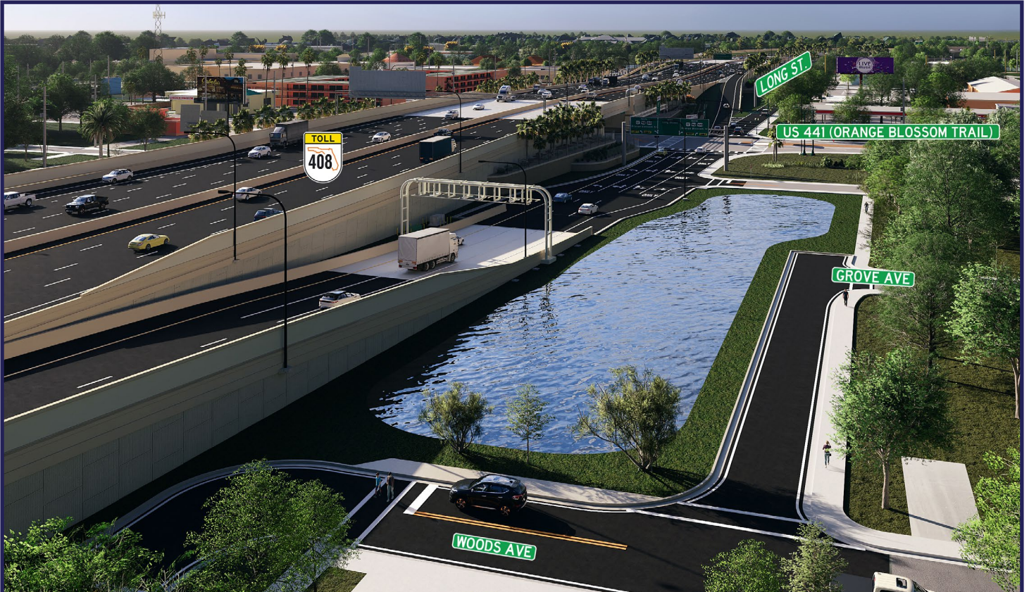
View of the westbound SR 408 off-ramp to US 441 (S. Orange Blossom Trail) showing the new stormwater management pond with a new one-way connection between Grove Avenue and Woods Avenue
