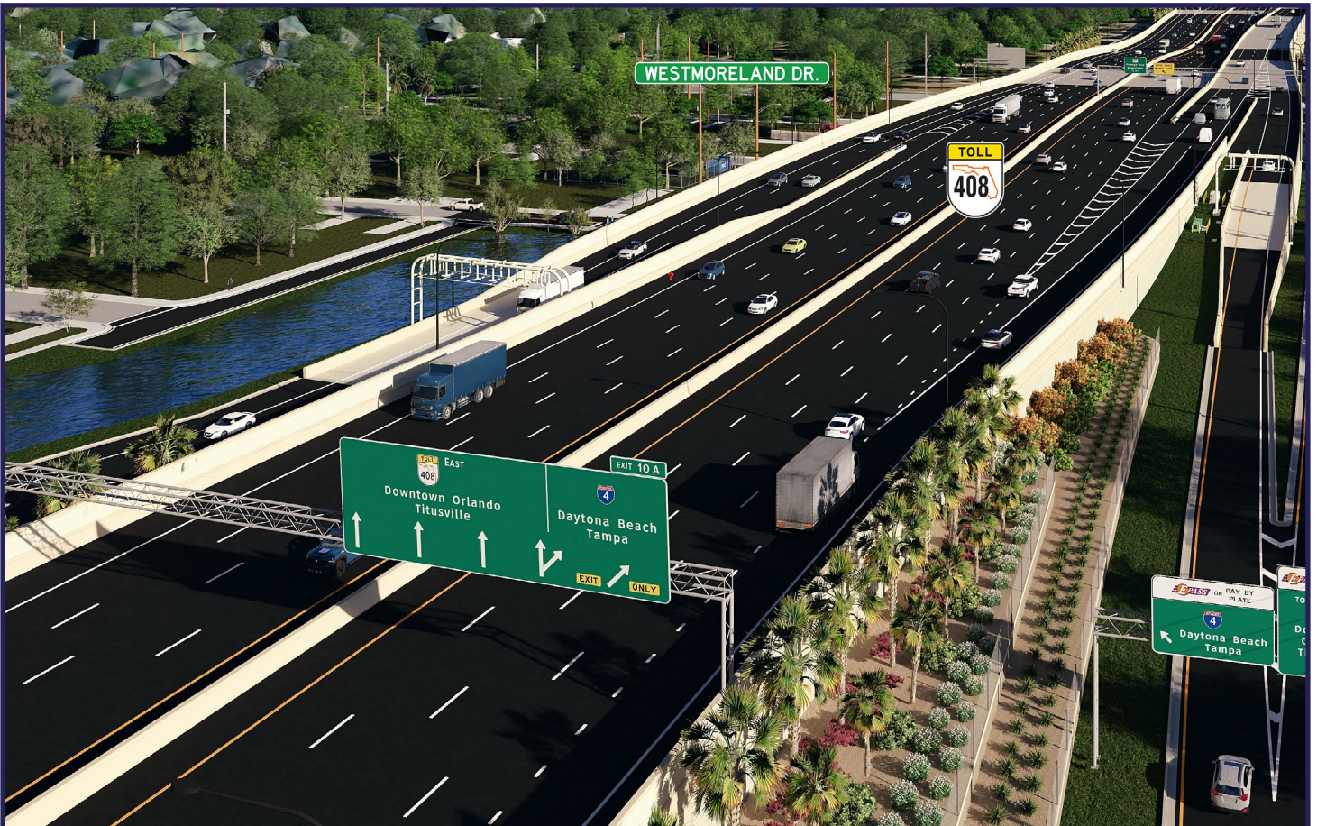
View of the new stormwater management pond from SR 408
