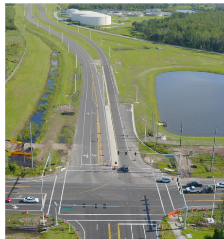
Realigned intersection of Poinciana Parkway and Cypress Parkway
