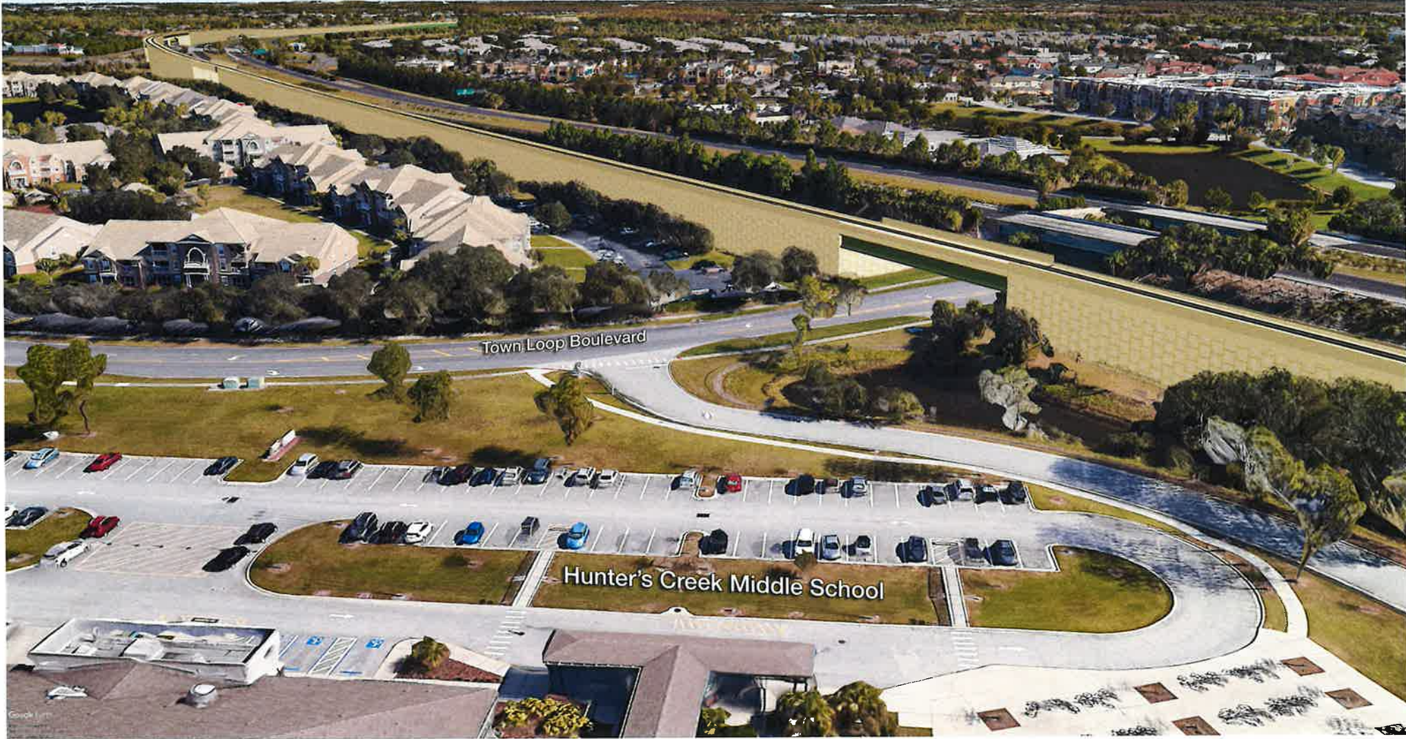
A view of the proposed Brightline Train's elevated wall as it runs adjacent to Hunter's Creek Middle School and crosses 30 feet above Town Loop Boulevard
