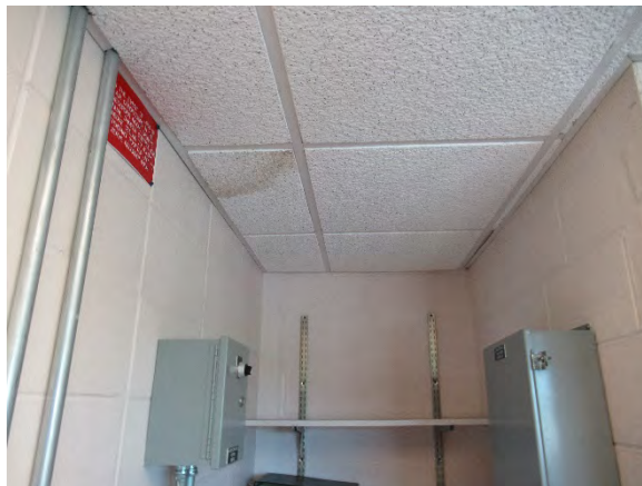
Figure 12: SR 417 Moss Park on ramp stained ceiling tile.
