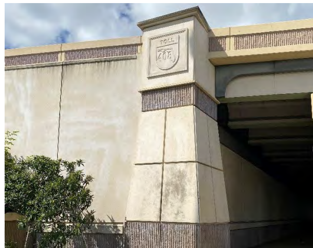
Figure 4: Discoloration on Architectural Column.
