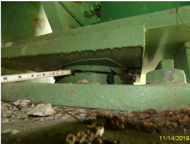
Figure 24: Extruded elastomer at Abutment bearings SR 417 over SR 528 bridge.
