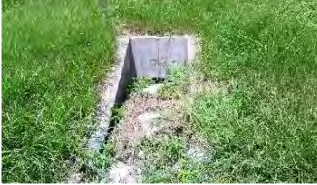
Figure 13: SR 429 obstructed drainage structure at Franklin Street.
