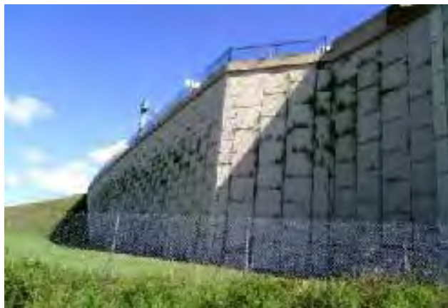
Figure 8: MSE wall vegetation FGT Gas Access Road.
