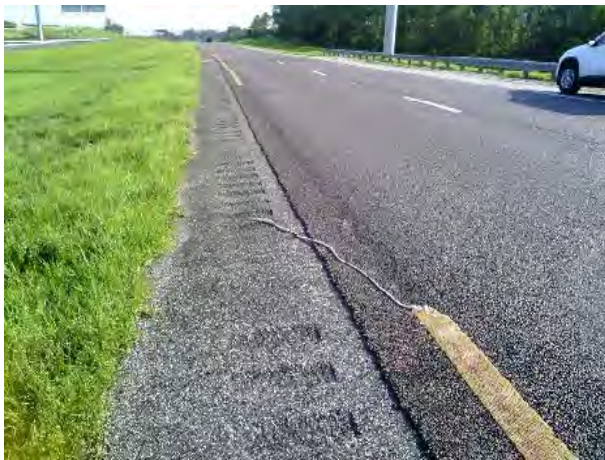
Figure 16: SR 451 damaged striping.
