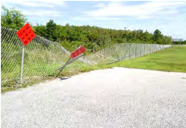
Figure 21: Damaged leaning fence on KOA Street.
