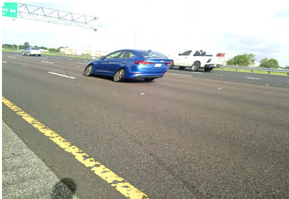
Figure 3: Pavement Marking Degradation east of Chickasaw Trail.
