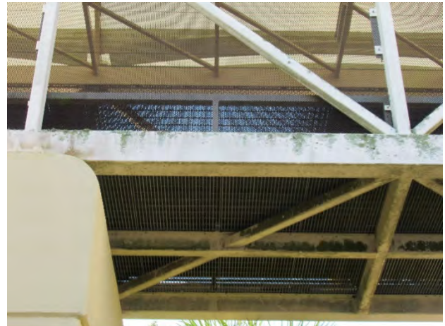
Figure 15: SR 429 Forest Lake Mainline Plaza mold growth on pedestrian bridge.
