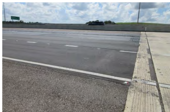
Figure 7: Spalling at expansion joint SR 414 over Landfill Service Road
