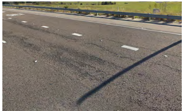
Figure 23: Asphalt Raveling and Cracking SR 414.
