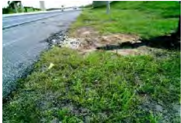
Figure 6: Roadside erosion SR 414.
