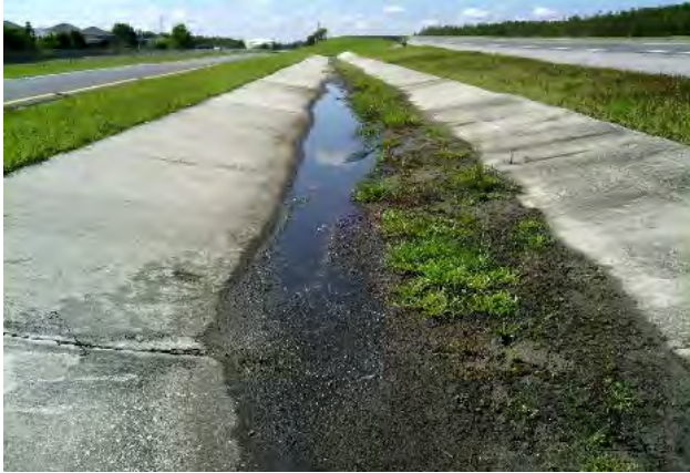
Figure 20: SR 538 sediment in ditch pavement west of KOA Street.
