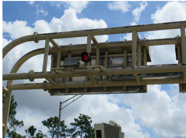
Figure 19: Toll Gantry with mold growth SR 528 Dallas Boulevard on ramp
