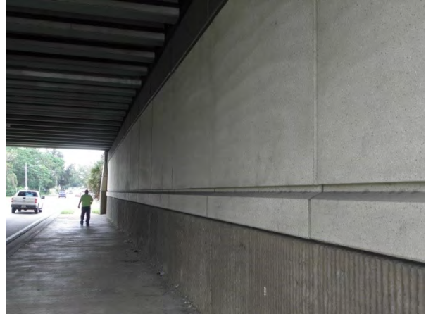
Figure 22: Cladding wall coating degradation SR 408.
