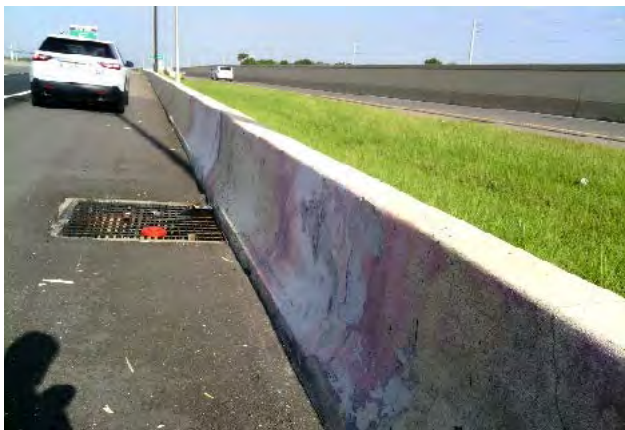
Figure 18: SR 528 barrier wall coating damage east of Boggy Creek Road.
