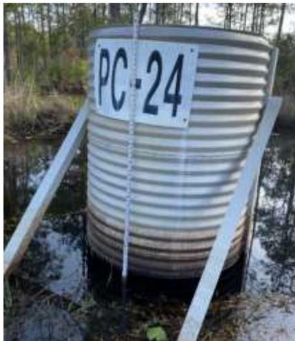
**PLATE 4. WEIR PC-24 AT THE INLET OF C-35**
