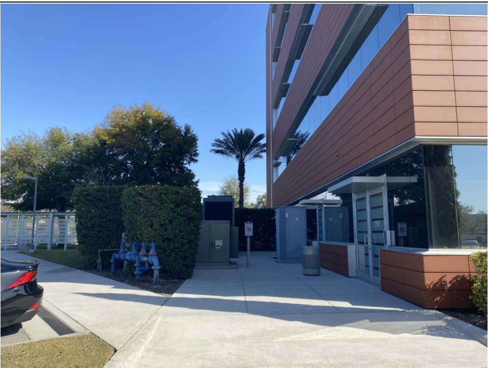
View of the emergency generator, belly tank, and pad-mounted electrical transformer, located on the northwest corner of the office building.
