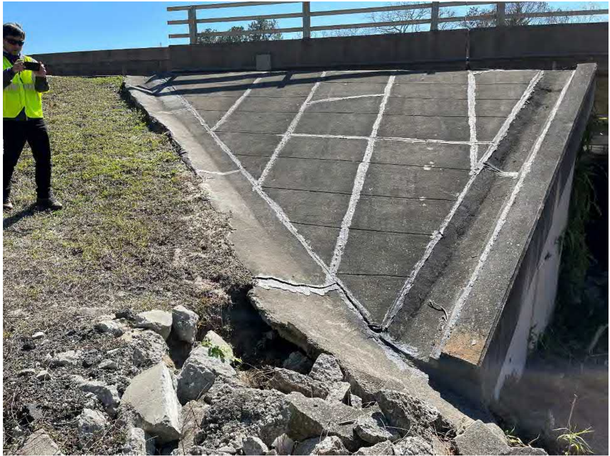
Erosion shown at Little Wekiva Canal Bridge near Lake Lotus Park Entrance
