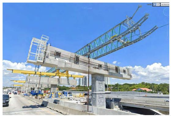
Figure 3. Beam Launcher with Temporary Post-Tensioning in Pier Cap (Ex. I-395 DB)
