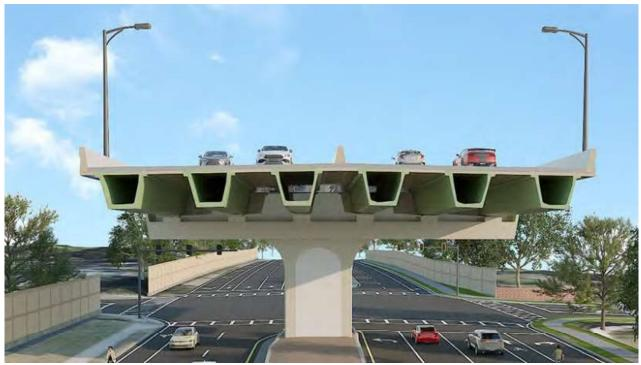
Figure 5A. B1 Typical Section (Br. XXXXXX) SR 414 Viaduct
