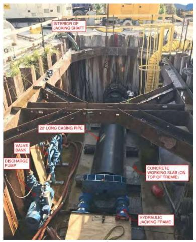
Figure 8. Example Jack and Bore Pit (similar to RCW relocation need)
