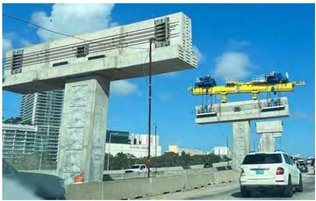
Figure 4. Precast Wing Lifter and Temporary Post-Tensioning in Pier Cap (Ex. I-395 DB)
