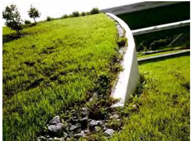
Figure 14: SR 429 wall gutter full of debris at Ponkan Road.
