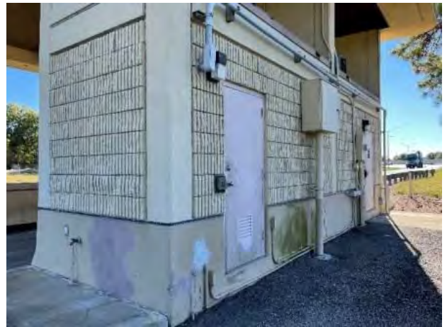
Figure 12: SR 417 Colonial off ramp coatings degradation.
