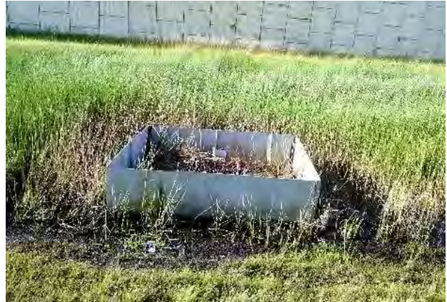
Figure 17: Overgrown weir structure SR 528 and Narcoossee Road.
