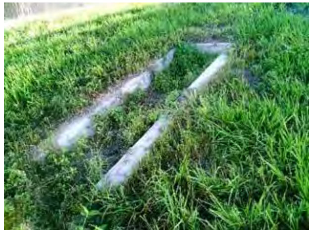
Figure 6: Overgrown mitered end section Coral Hills Mainline Plaza Pond.
