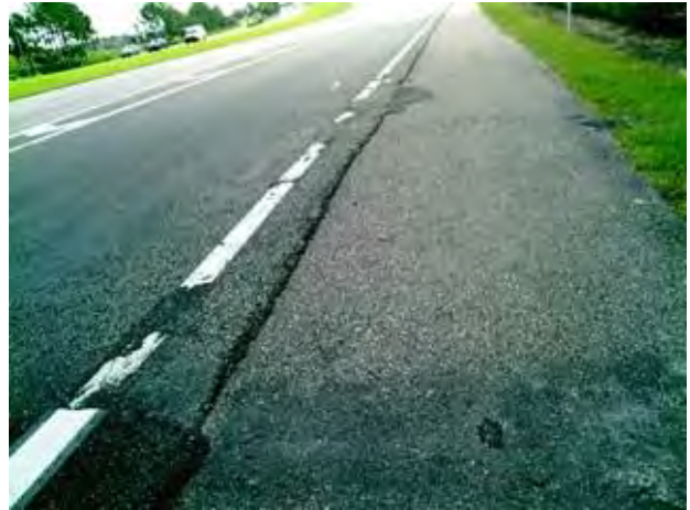
Figure 13: SR 429 pavement marking degradation CR 535 off ramp.
