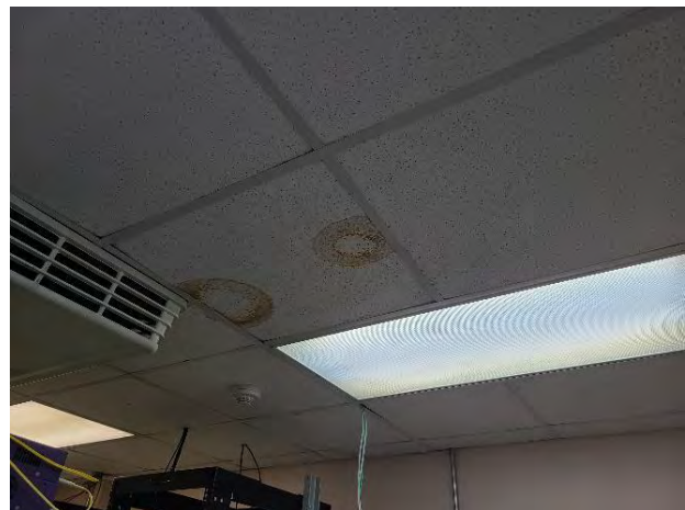
Figure 19: Water damaged ceiling tile Beachline Main Plaza.
