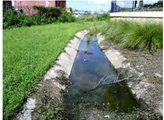
Figure 3: Flume drainage structure needs vegetation cleared.
