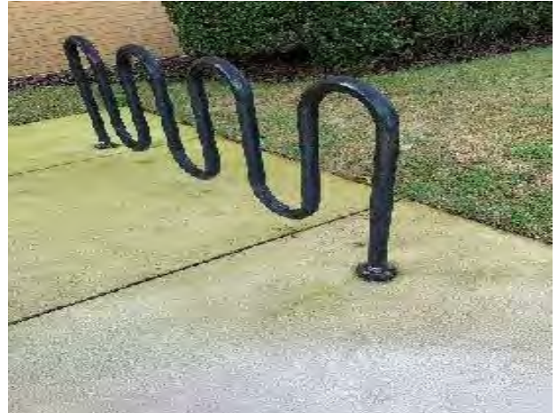
Figure 20: CFX Administration and Operations Building sidewalk with dirt and algae growth.
