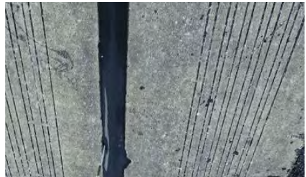
Figure 4: Joint sealant degradation SR 408 over Andes Road.
