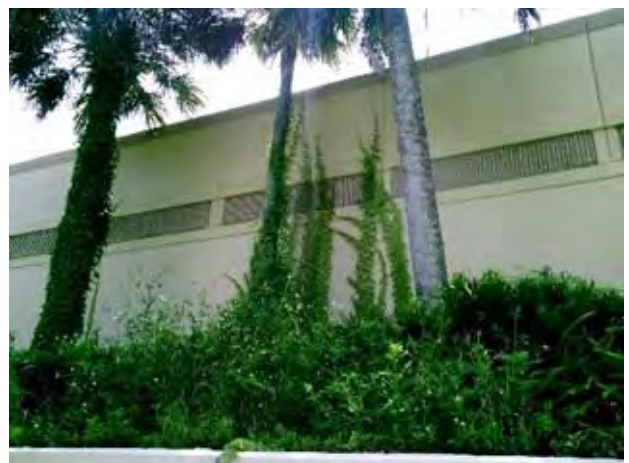
Figure 5: Vegetation of Noise Wall at SR 408 and Mills
