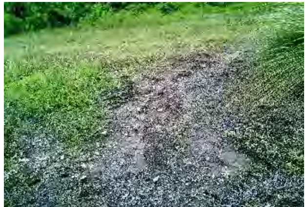
Figure 10: Minor bed erosion at International Drive
