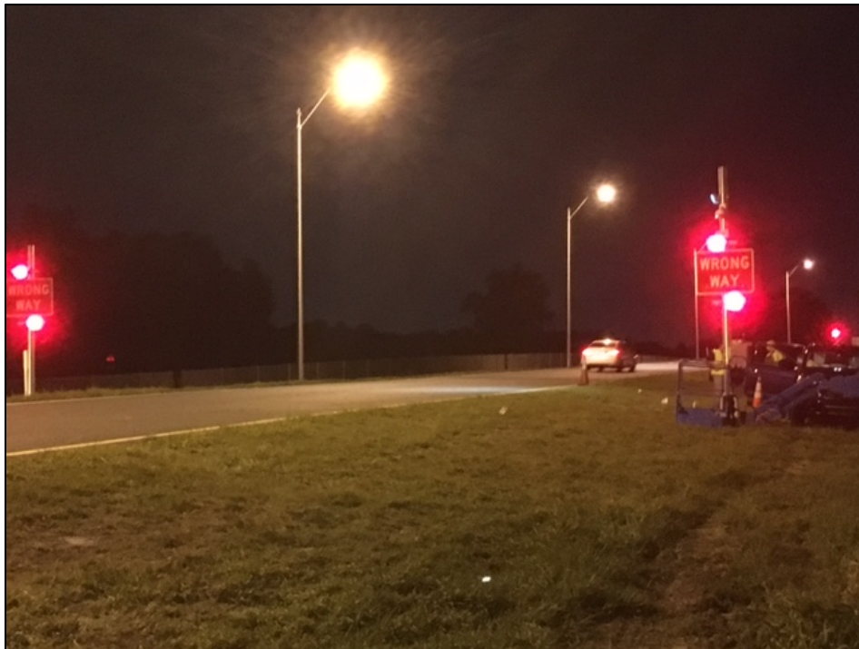
Figure 10.5: Wrong Way Driving Installation Testing
