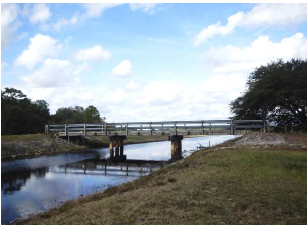
Figure 2.20.1: Bridge over C-32C Canal (Looking North)
