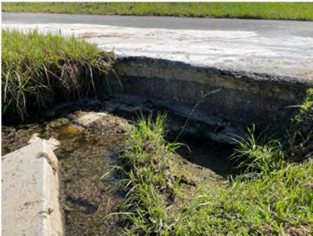
15" Drop off on Binion Road (facing east)
