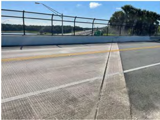
Pavement seam and approach slab on South side of Binion Rd Bridge (facing east)
