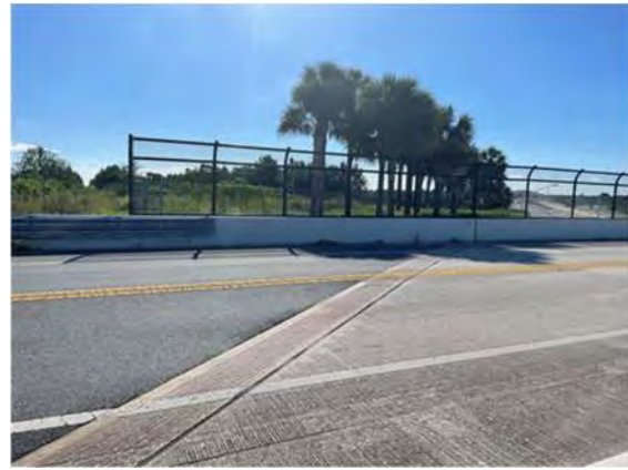
Pavement seam and approach slab on North side of Binion Rd Bridge (facing east)
