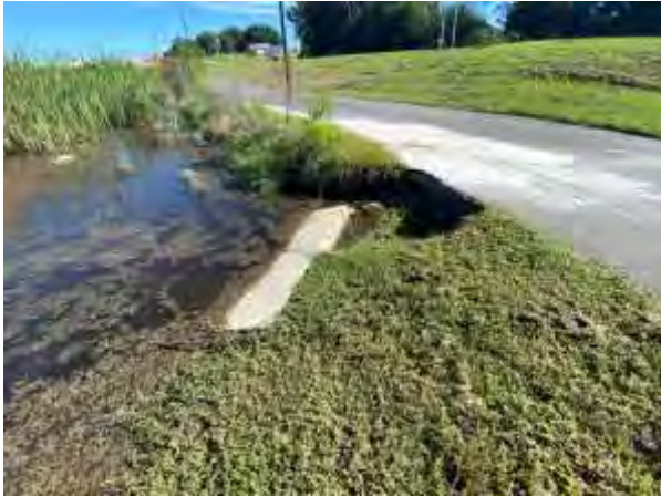
Ponding and Erosion at outfall of shared-used path inlet near Binion Rd cross drain (facing north)
