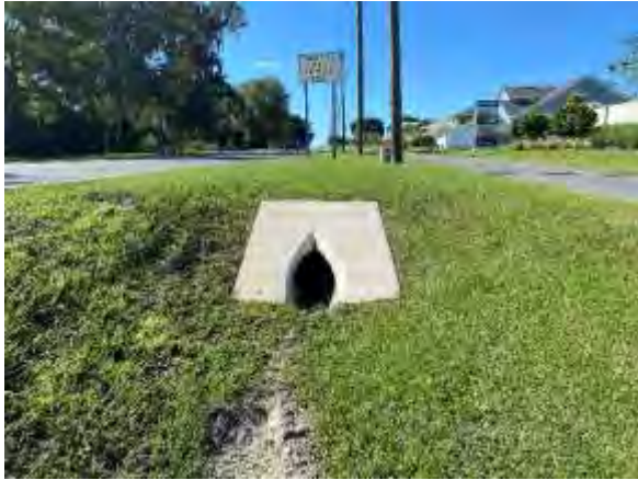
MES for side drain along Binion Rd at the Winterstone St Intersection (facing south)
