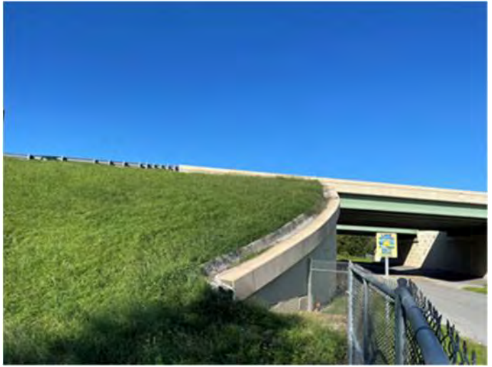
Gutter behind Retaining Wall (facing east)
