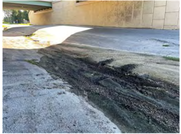
Erosion under Lust Rd Bridge (facing east)
