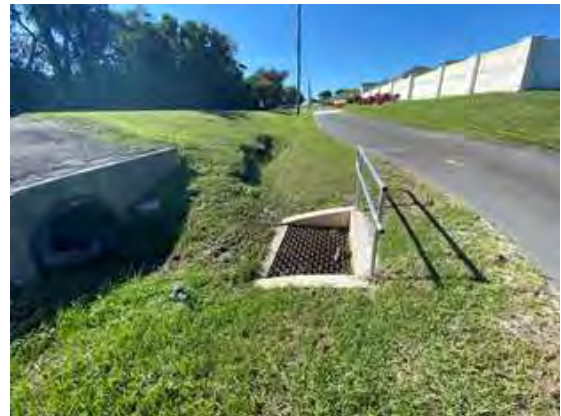
Binion Rd cross drain headwall (left) and inlet along shared-used path (right) (facing south)
