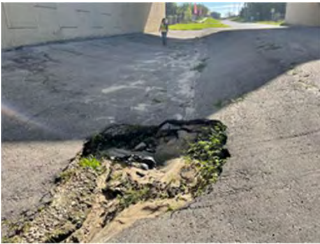
Pothole in shoulder under Lust Rd Bridge (facing east)
