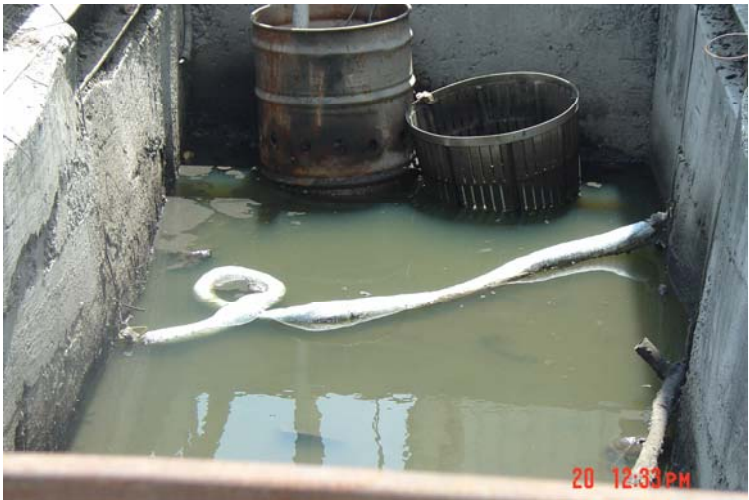
Fig. 9 & 10-Storm water oil water separators.
