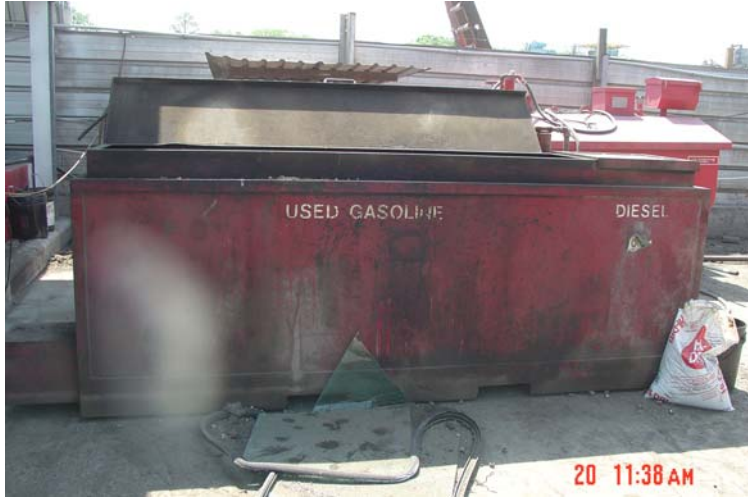
Fig. 1 & 2-Aboveground storage tank larger than 550-gallons.
