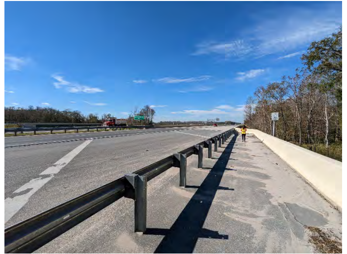
SR 528 Bridge over Econ River (facing west)
