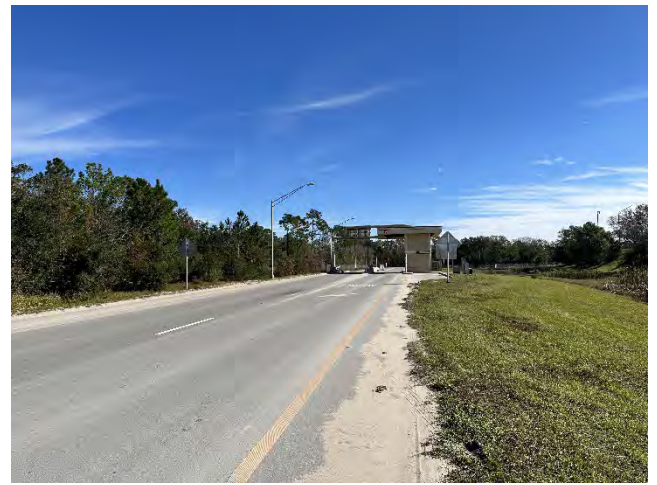
Backside of SR 528 On-Ramp at Dallas Blvd (facing east)
