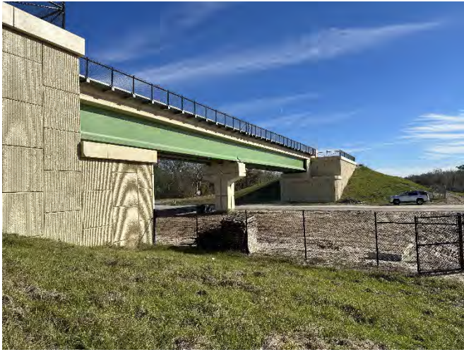
Brightline Bridge over Dallas Blvd (facing northeast)
