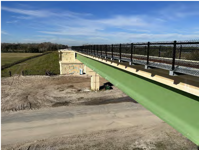
Brightline Bridge over Dallas Blvd (facing west)
