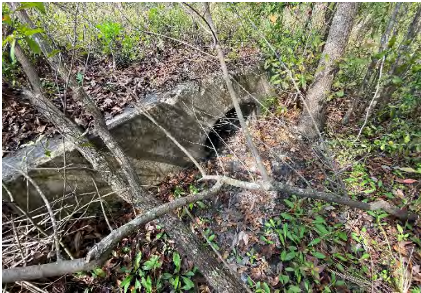
Upstream of 19" x 45" ERCP crossing Dallas Blvd just north of the on-ramp. (Facing northwest)
