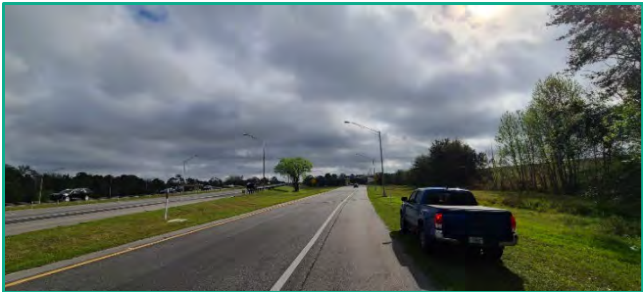
Figure 9 - Westbound On-Ramp Lighting
