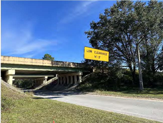
SR 528 Bridges over Dallas Blvd (facing south)
