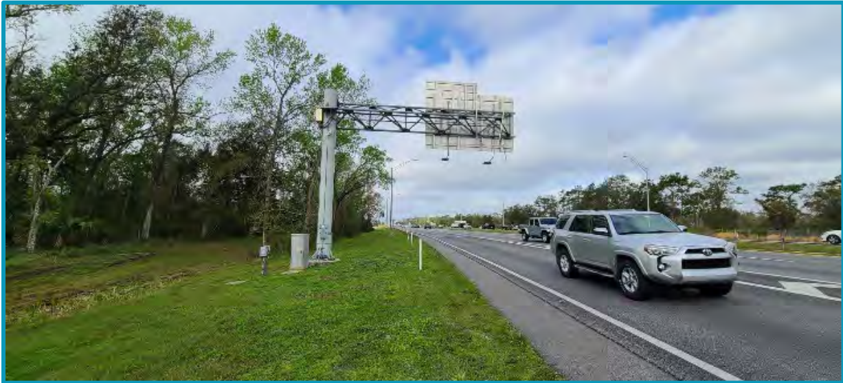
Figure 10 - Eastbound Off-Ramp Sign Fixtures
