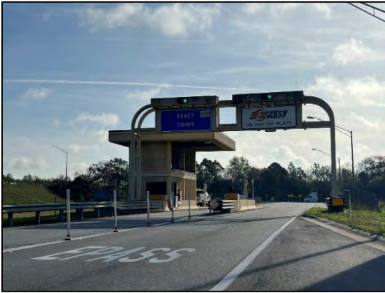
Figure 22 - Toll Plaza - Eastbound Exit
