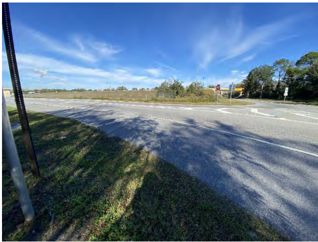
SR 528 Eastbound Exit Intersection with Dallas Blvd (facing north)
