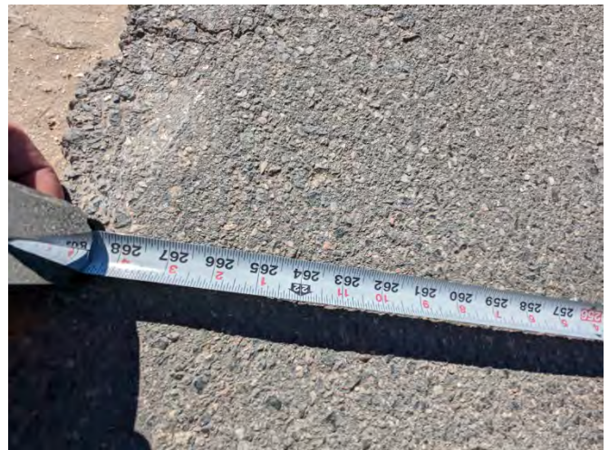
22'6" (270") pavement width of Dallas Blvd under SR 528 Bridges
