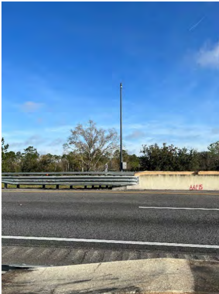
Figure 20 - Device 10 (CCTV, MM 23.8)
