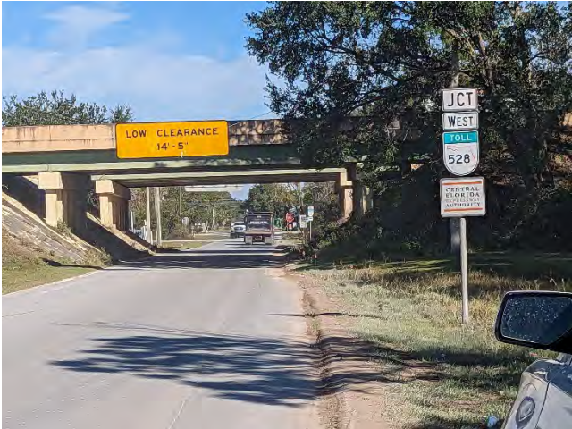
SR 528 Bridges over Dallas Blvd (facing north)
