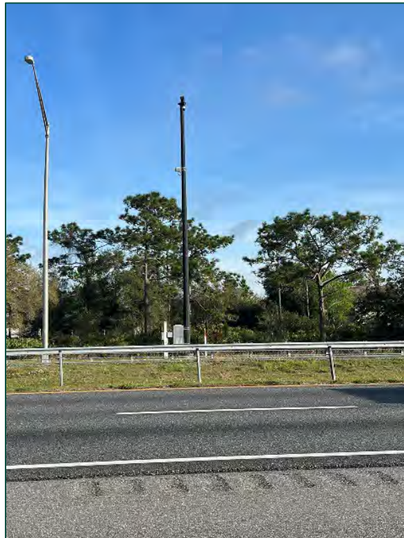
Figure 17 - Devices 6 & 7 (CCTV and TMS, MM 23.3)
