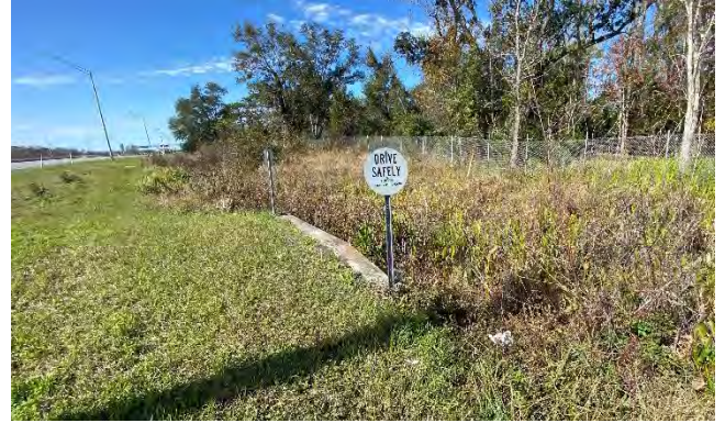
Upstream of 36" RCP Cross Drain at Station 1444+00 BL SR 528. (facing northeast)
