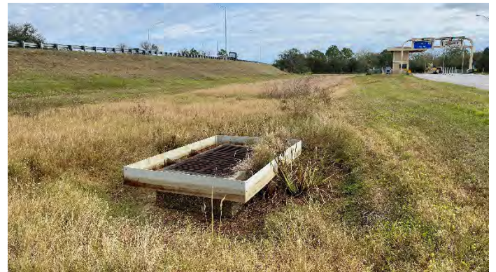
Pond 403-1B and control structure within the infield of the existing off-ramp and SR 528 eastbound. Vegetation in skimmer. (facing east)
