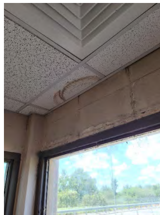
Figure 36 CR-535 Ramp On
