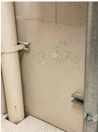
Figure 45 Lake Nona Ramp On
