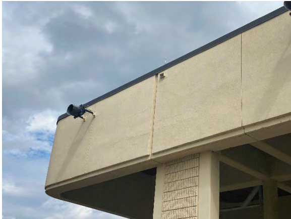
Figure 25 South Access Ramp Off
