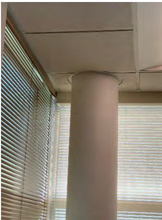
Figure 41 Building Headquarters Second Floor (Room 235)
