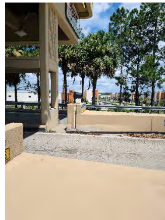
Figure 18 SR-438 Ramp Off
