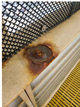
Figure 4 Pine Hills Mainline
