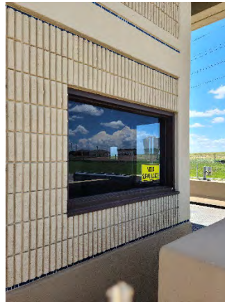
Figure 22 New Independence Ramp On
