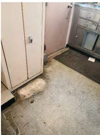
Figure 11 Colonial Ramp Off
