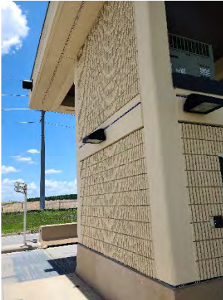
Figure 21 New Independence Ramp On
