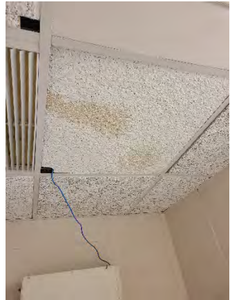
Figure 48 Mills Ramp Off
