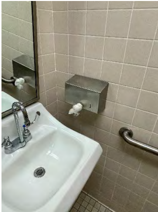
Figure 13 Pine Hills Mainline
