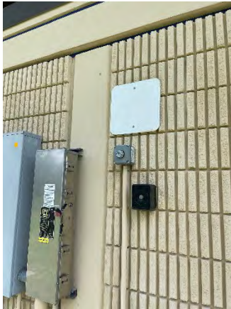
Figure 45 Dallas Ramp On
