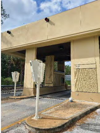
Figure 49 Hiawassee Ramp On
