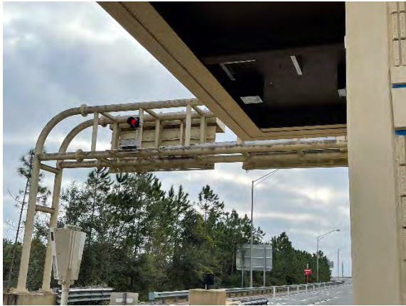
Figure 13 Keene Road Ramp Off
