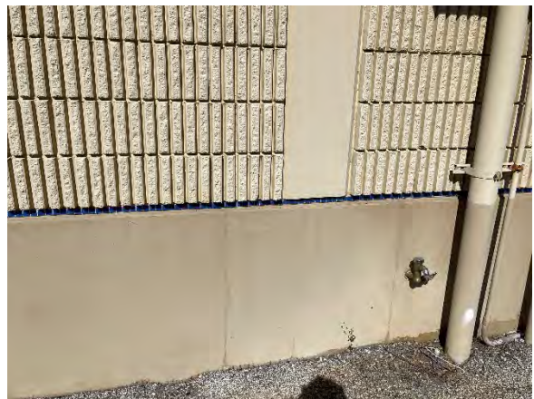
Figure 28 South Access Ramp Off
