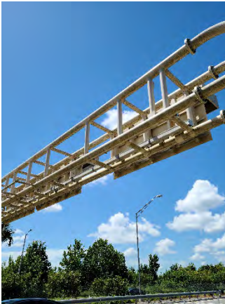
Figure 33 CR-535 Ramp On
