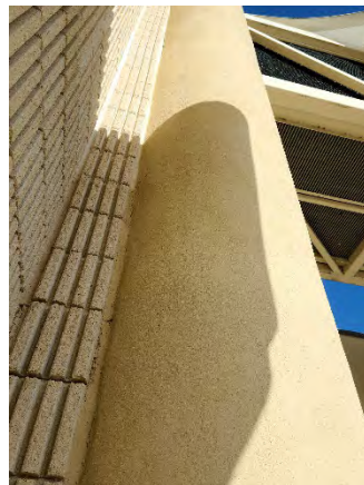
Figure 12 Coral Hills Mainline
