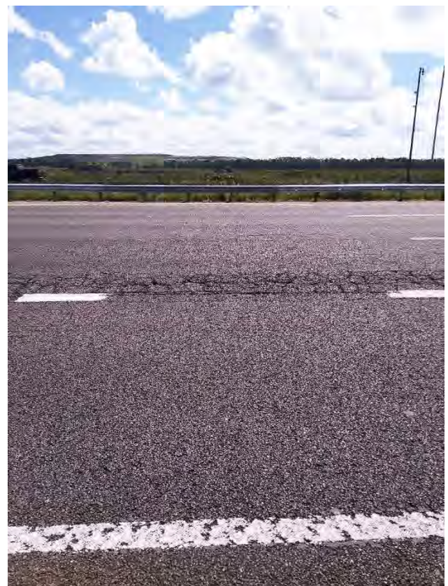
Figure 10: Pavement and pavement markings
