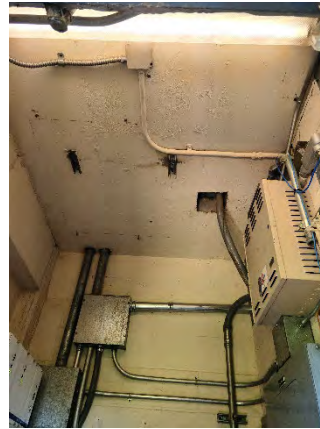
Figure 14 Colonial Ramp Off
