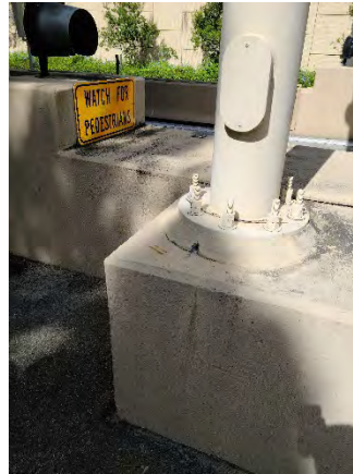
Figure 16 Keene Road Ramp On
