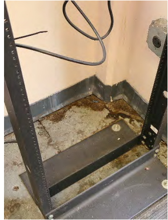
Figure 46 Mills Ramp Off
