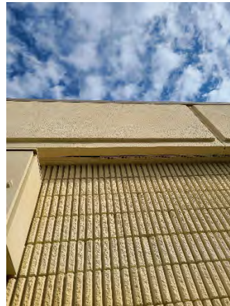
Figure 14 Boggy Creek Mainline
