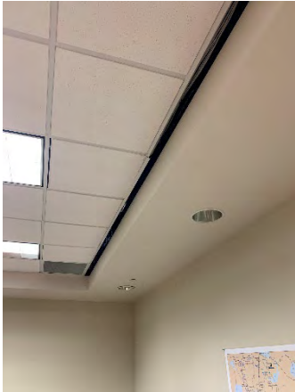
Figure 19 Building Headquarters First Floor (Room 136)
