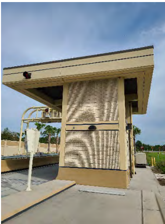
Figure 17 Rouse Road Ramp Off
