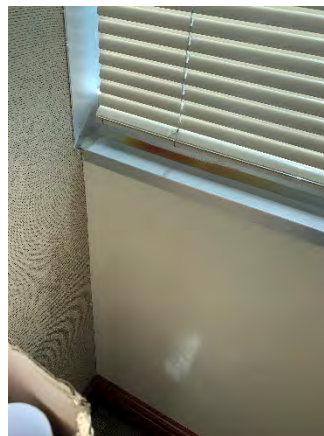
Figure 60 Building Headquarters Third Floor (Room 347)
