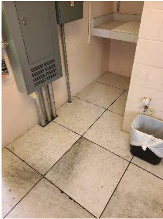
Figure 31 Conway Ramp On
