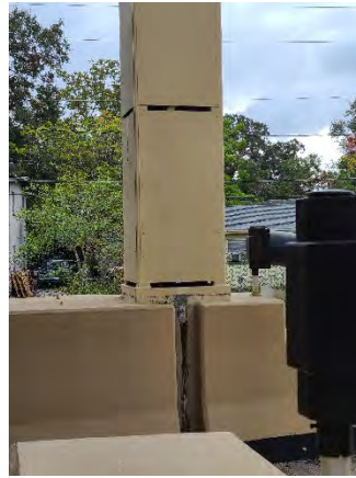
Figure 38 OB T Ramp On
