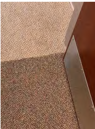
Figure 35 Building Headquarters Second Floor (Room 223)
