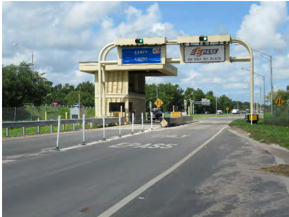
Figure 43 Dallas Ramp On
