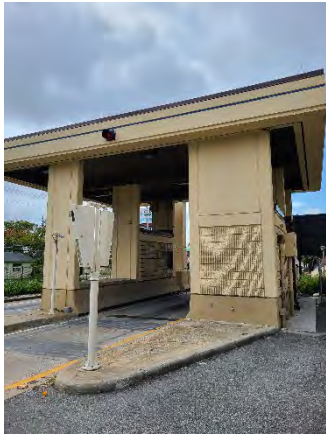
Figure 37 OB T Ramp On
