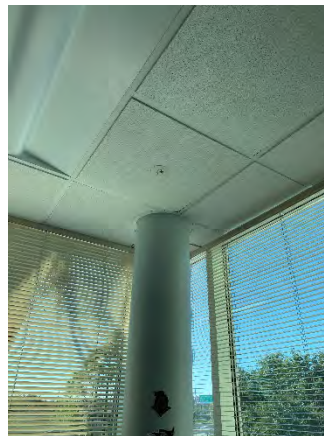
Figure 42 Building Headquarters Second Floor (Room 235)
