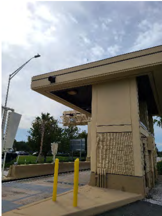
Figure 19 Rouse Road Ramp On
