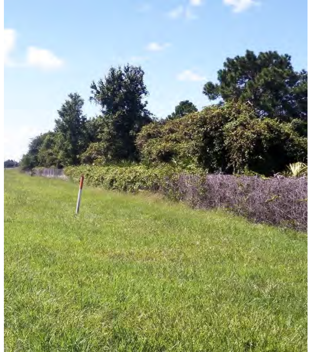
Figure 11: Overgrown fence - SR 417
