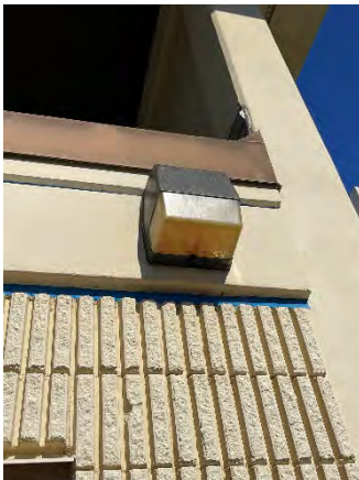
Figure 35 Good Homes Ramp On
