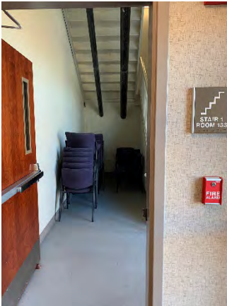
Figure 27 Building Headquarters First Floor (Stair 133)
