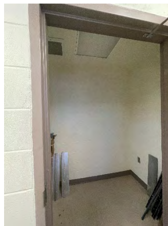
Figure 48 Conway Ramp Off
