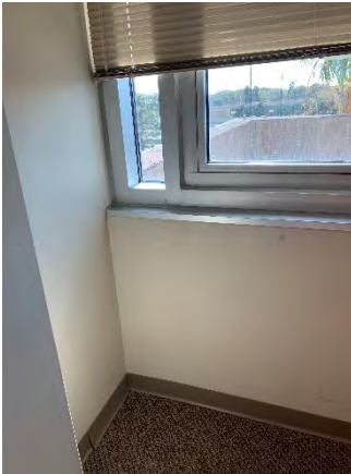
Figure 51 Building Headquarters Third Floor (Room 356)
