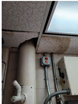
Figure 28 Landstar Ramp Off
