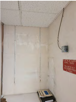
Figure 41 Good Homes Ramp Off
