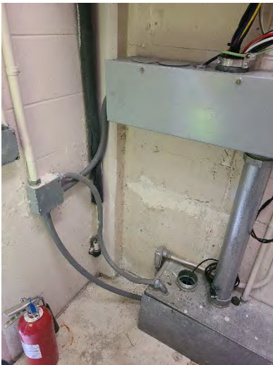
Figure 47 Hiawassee Ramp Off
