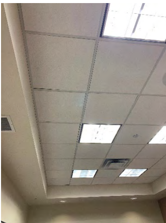
Figure 11 Building Headquarters First Floor (Room 148)
