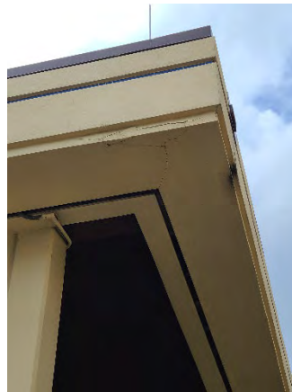
Figure 40 OB T Ramp On
