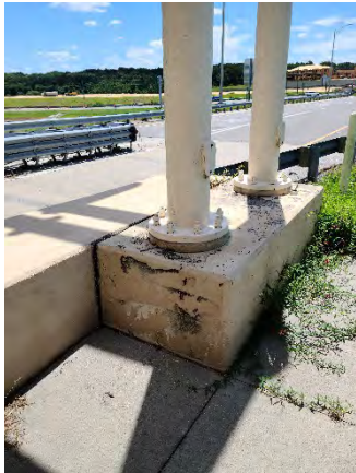
Figure 31 CR-437A Ramp On
