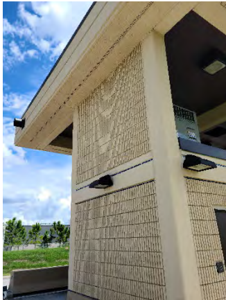
Figure 25 New Independence Ramp Off
