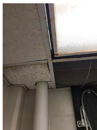
Figure 6 Boggy Creek Mainline
