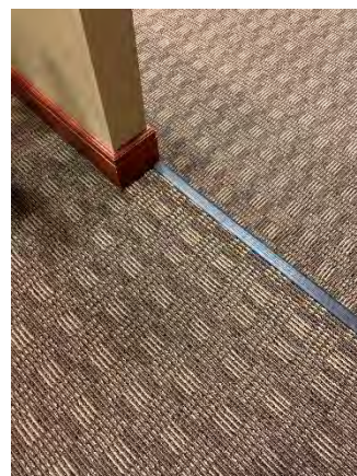
Figure 30 Building Headquarters First Floor (Board room 156)
