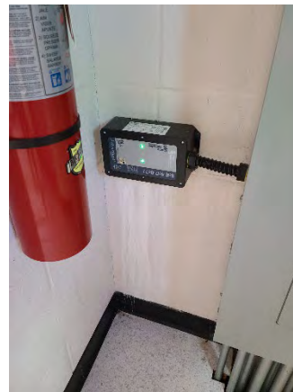
Figure 30 CR-437A Ramp On
