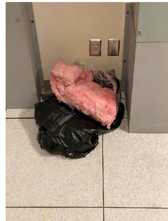
Figure 70 Moss Park Ramp On
