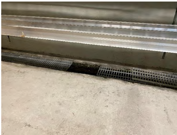
Figure 9 Boggy Creek Mainline
