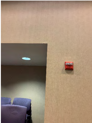
Figure 31 Building Headquarters First Floor (Board room 156)
