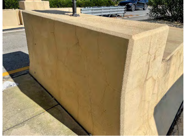
Figure 36 Good Homes Ramp On
