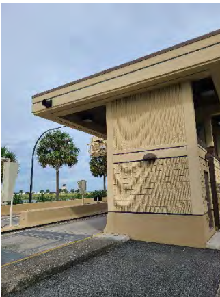
Figure 29 Conway Ramp On
