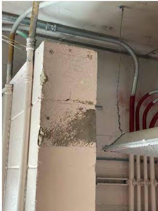
Figure 43 Lake Nona Ramp On
