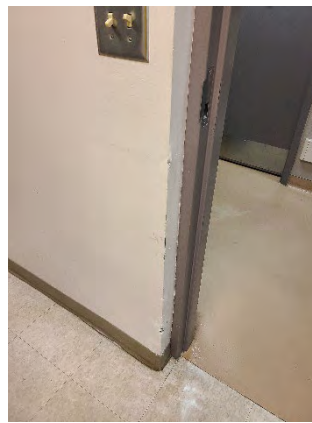
Figure 10 Pine Hills Mainline
