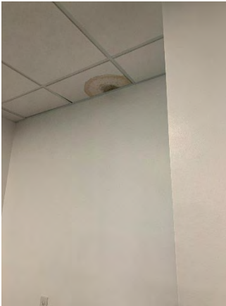
Figure 39 Building Headquarters Second Floor (Room 239)
