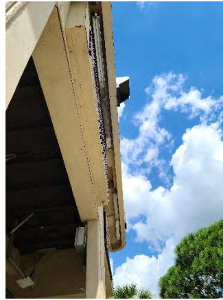
Figure 20 US-441 Ramp On
