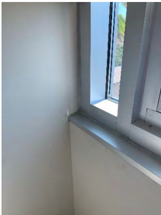
Figure 53 Building Headquarters Third Floor (Room 356)
