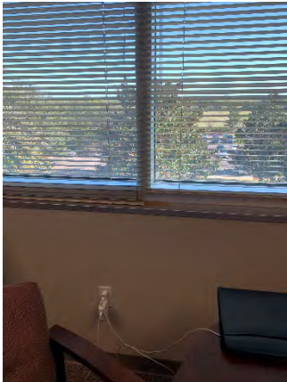
Figure 55 Building Headquarters Third Floor (Room 33)
