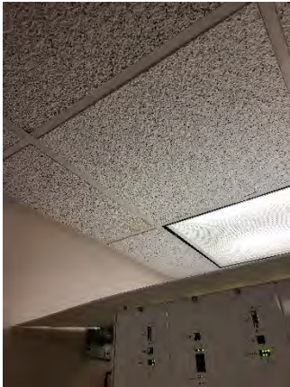
Figure 7 Pine Hills Mainline
