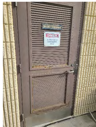
Figure 16 Boggy Creek Mainline
