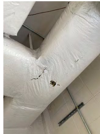
Figure 64 Moss Park Ramp Off
