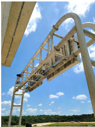
Figure 29 CR-437A Ramp On
