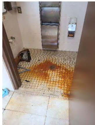
Figure 24 John Young Parkway Ramp Off
