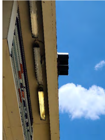
Figure 20 West Road Ramp On
