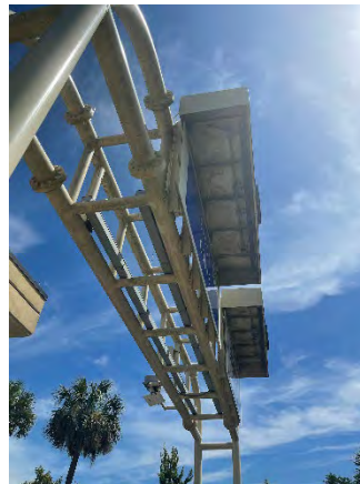
Figure 46 Conway Ramp Off
