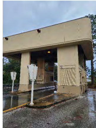
Figure 44 Hiawassee Ramp Off
