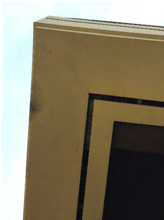
Figure 39 OB T Ramp On
