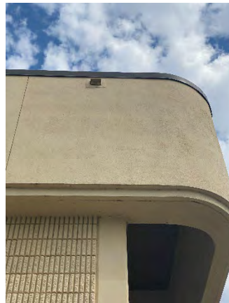
Figure 26 South Access Ramp Off
