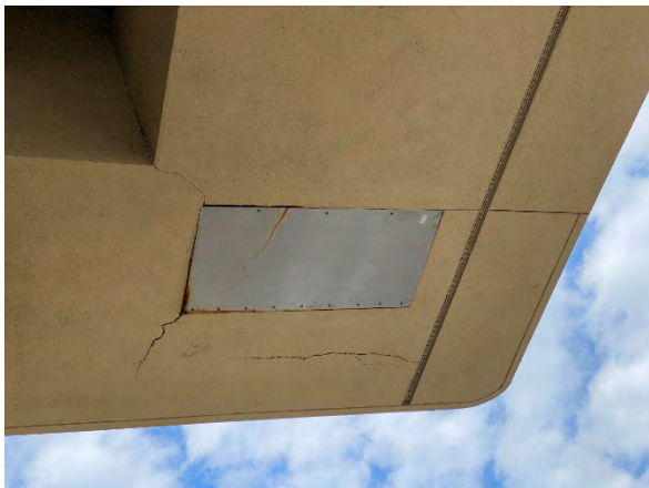
Figure 11 Boggy Creek Mainline
