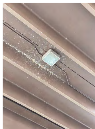
Figure 12 Boggy Creek Mainline
