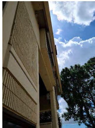
Figure 14 US-441 Ramp Off
