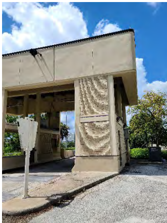
Figure 27 Landstar Ramp Off
