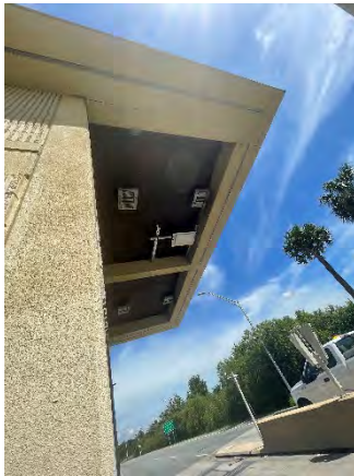
Figure 45 Conway Ramp Off
