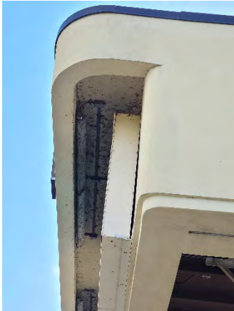
Figure 7 Coral Hills Mainline
