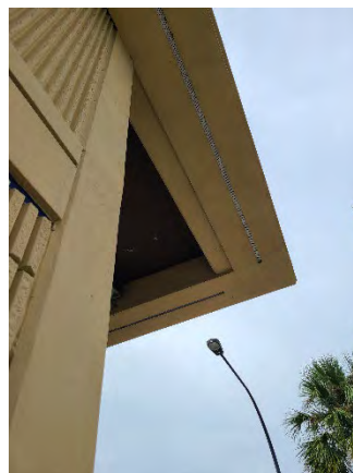
Figure 30 Conway Ramp On
