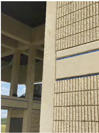
Figure 27 South Access Ramp Off
