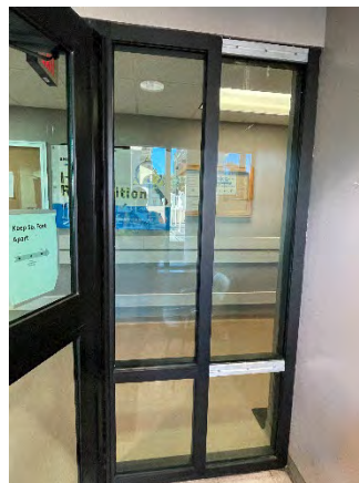
Figure 12 Pine Hills Mainline
