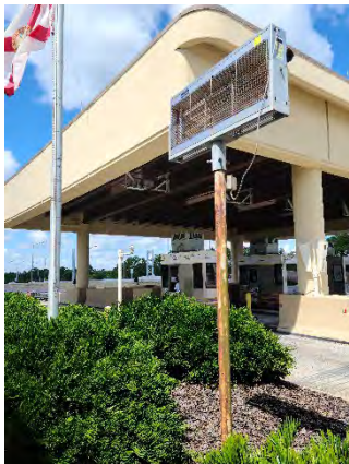
Figure 5 John Young Pkwy Mainline
