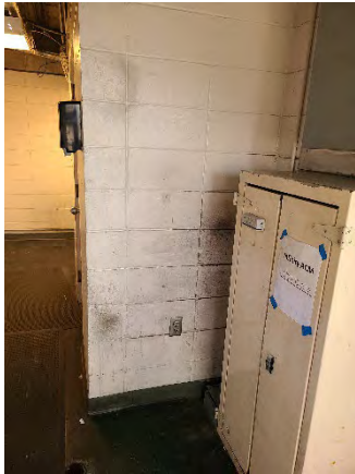
Figure 41 OB T Ramp On
