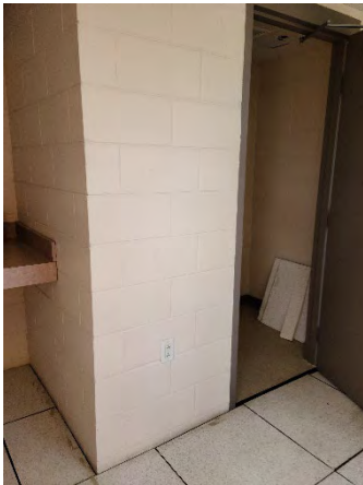
Figure 27 New Independence Ramp Off
