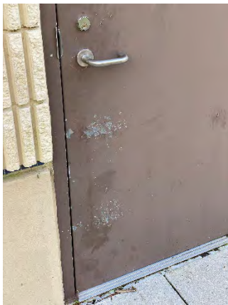
Figure 41 Lake Nona Ramp On
