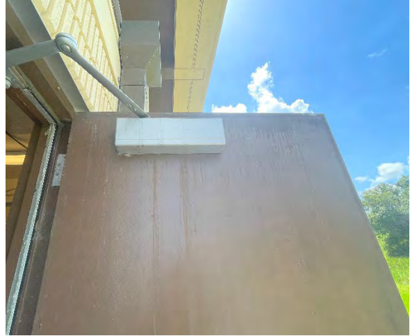
Figure 50 Dallas Ramp On
