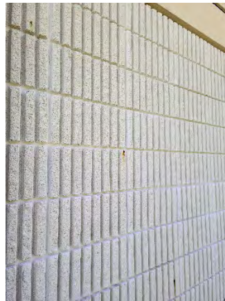
Figure 14 Schofield Ramp On
