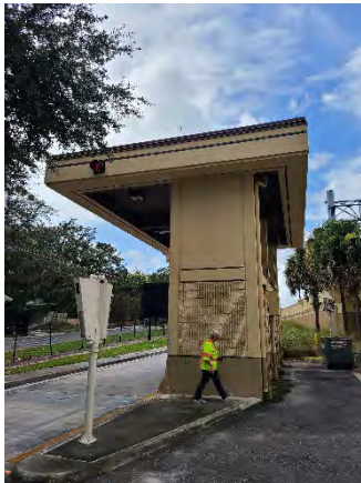
Figure 45 Mills Ramp Off
