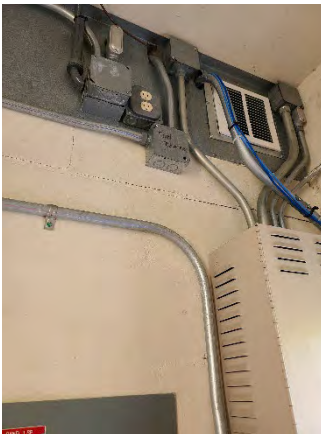
Figure 23 Rouse Road Ramp On
