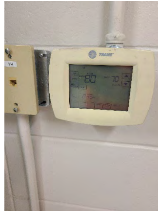
Figure 38 Good Homes Ramp On
