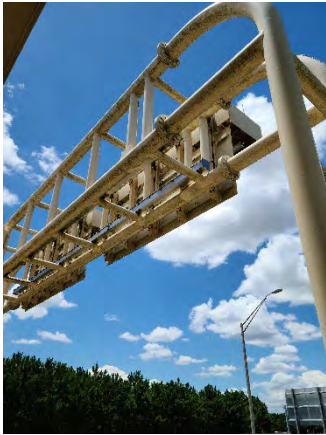
Figure 13 Schofield Ramp On
