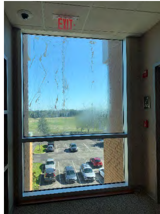
Figure 50 Building Headquarters Third Floor (Room 312)
