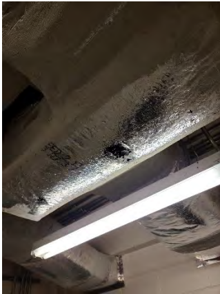
Figure 19 Schofield Ramp Off
