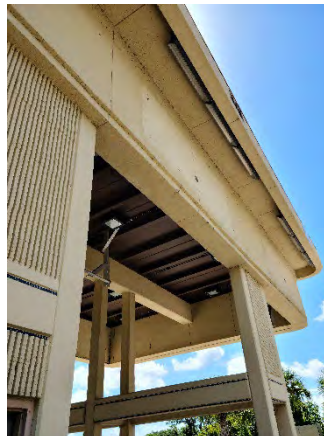
Figure 34 CR-535 Ramp On
