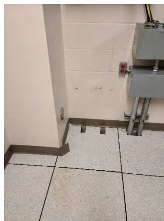
Figure 16 Schofield Ramp On
