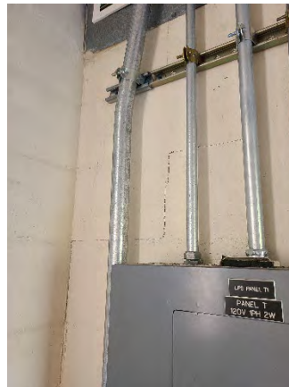
Figure 24 Rouse Road Ramp On
