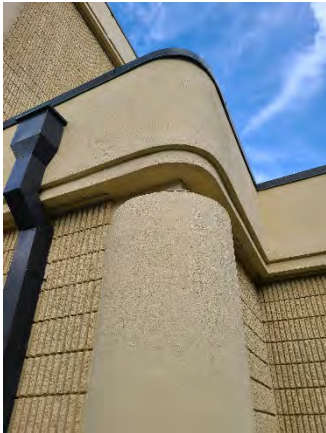
Figure 1 Pine Hills Mainline
