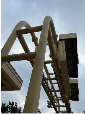
Figure 19 Hiawassee Ramp On
