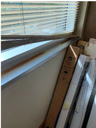
Figure 59 Building Headquarters Third Floor (Room 347)
