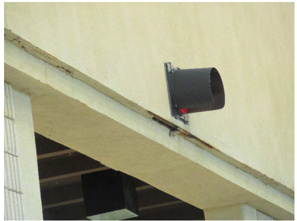
Figure 10 Coral Hills Mainline
