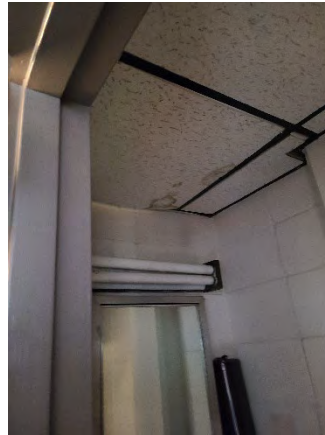
Figure 42 OB T Ramp On
