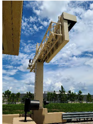
Figure 26 New Independence Ramp Off
