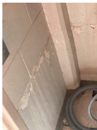
Figure 30 South Access Ramp Off
