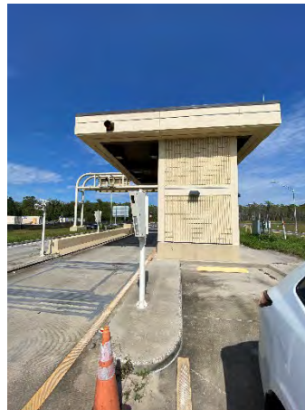
Figure 60 Moss Park Ramp Off
