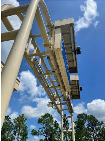
Figure 49 Dallas Ramp On
