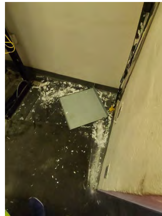
Figure 34 Conway Ramp Off
