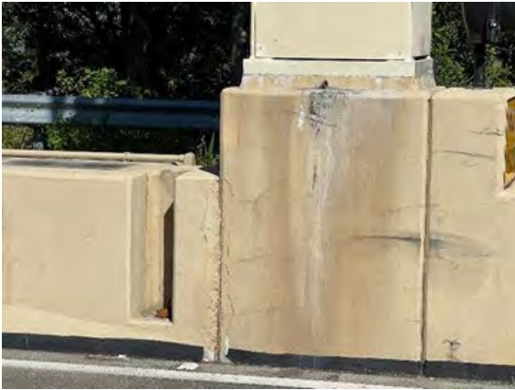
Figure 39 Good Homes Ramp Off
