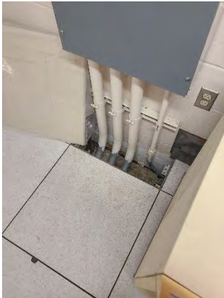
Figure 43 Good Homes Ramp Off
