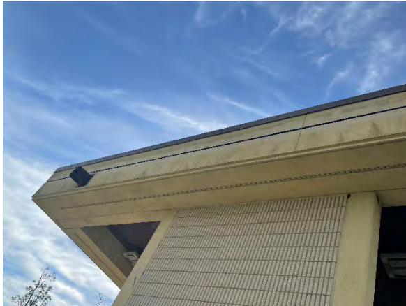
Figure 61 ICP Ramp Off
