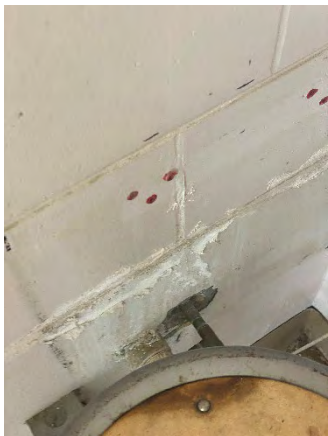
Figure 29 South Access Ramp Off
