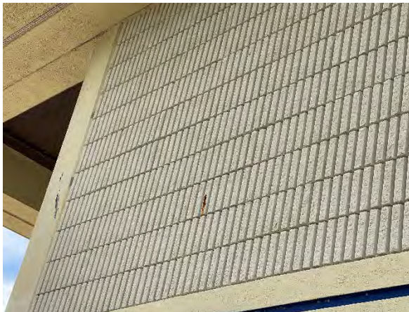
Figure 65 ICP Ramp Off
