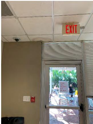
Figure 21 Building Headquarters First Floor (Break room)
