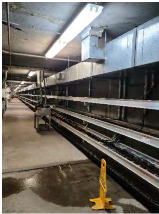
Figure 3 John Young Pkwy Mainline
