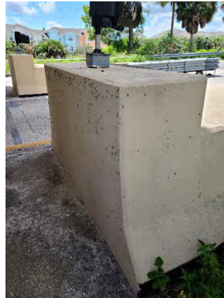
Figure 26 Landstar Ramp Off
