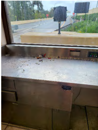
Figure 23 John Young Parkway Ramp Off
