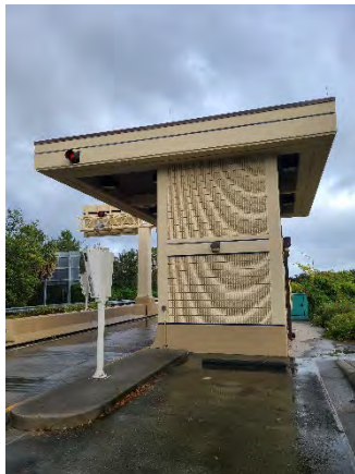
Figure 33 Good Homes Ramp On
