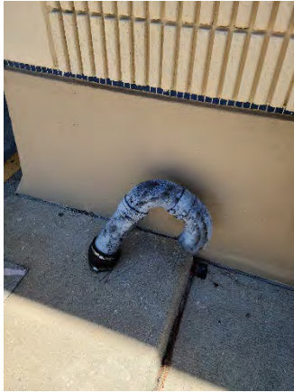
Figure 19 West Road Ramp On
