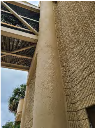
Figure 3 Pine Hills Mainline
