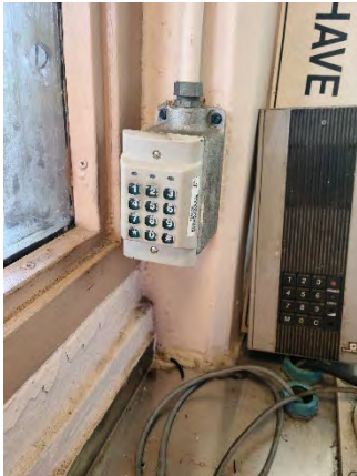
Figure 13 Colonial Ramp Off
