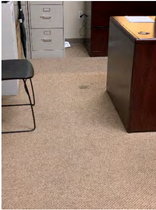
Figure 37 Building Headquarters Second Floor (Room 252)
