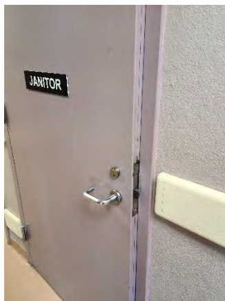
Figure 5 Coral Hills Mainline
