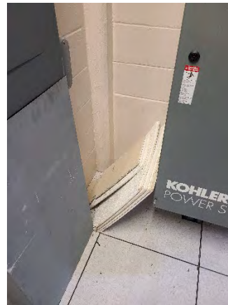
Figure 32 Conway Ramp On
