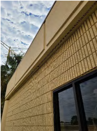
Figure 15 Boggy Creek Mainline
