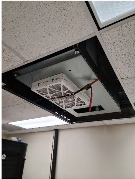
Figure 1 Coral Hills Mainline
