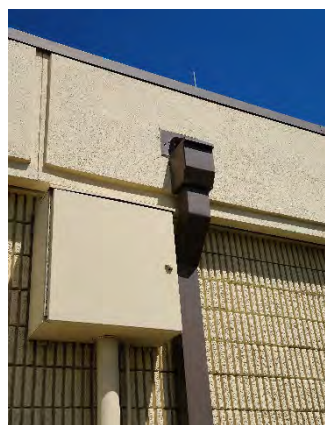
Figure 6 John Young Pkwy Mainline
