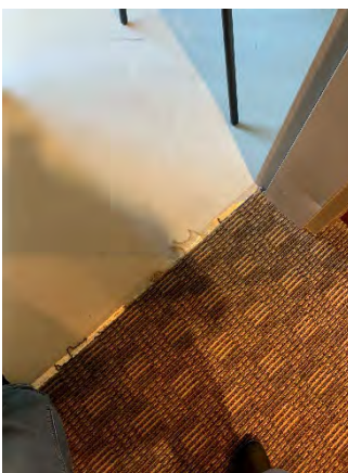
Figure 29 Building Headquarters First Floor (Board room 156)
