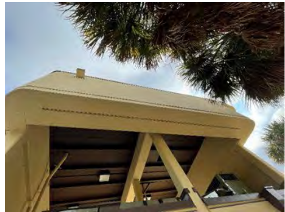
Figure 16 SR-438 Ramp Off
