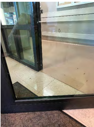
Figure 11 Pine Hills Mainline
