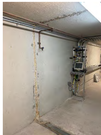
Figure 10 Boggy Creek Mainline
