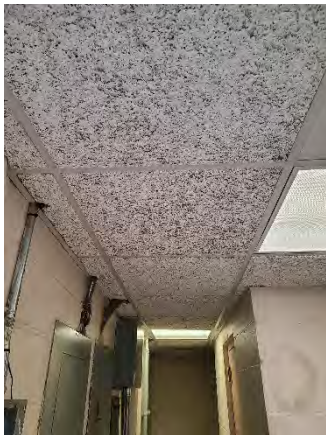
Figure 47 Mills Ramp Off
