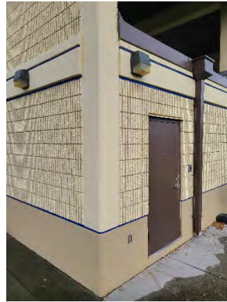
Figure 34 Good Homes Ramp On
