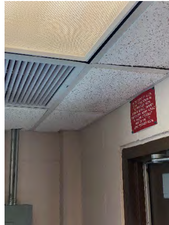
Figure 62 Moss Park Ramp Off
