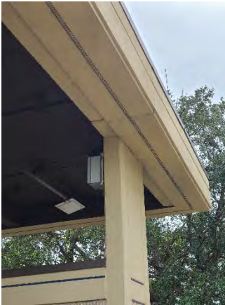
Figure 33 Conway Ramp Off
