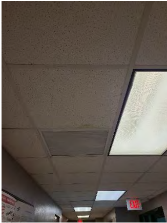
Figure 1 Conway EB Mainline
