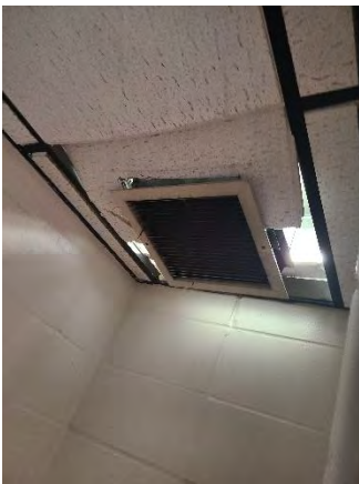
Figure 53 OB T Ramp Off
