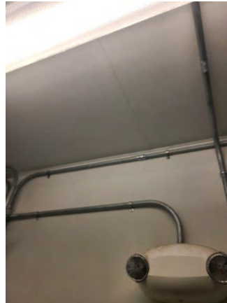
Figure 12 KOA AET Toll Plaza
