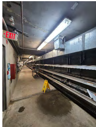
Figure 8 John Young Pkwy Mainline
