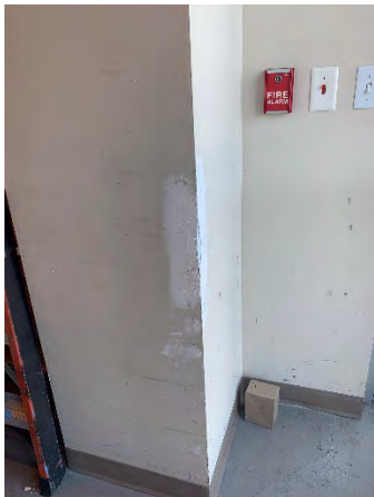
Figure 41 Building Headquarters First Floor (Room 132)
