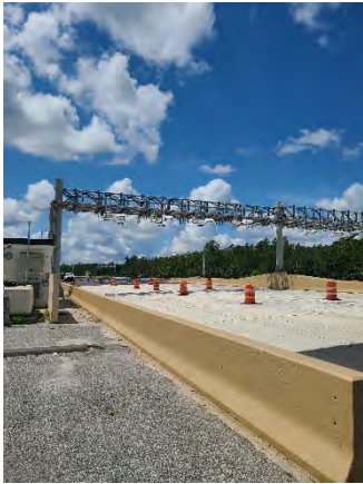
Figure 1 Marigold AET Toll Plaza
