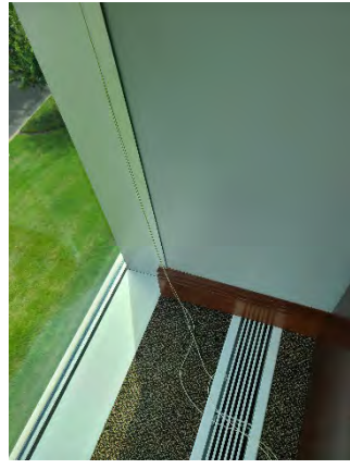
Figure 196 Building Headquarters Third Floor (Room 352D)
