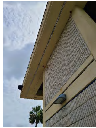
Figure 44 Conway Ramp Off
