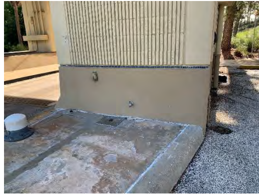
Figure 44 Hiawassee Ramp Off
