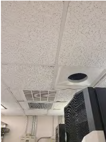
Figure 1 Forest Lake Mainline
