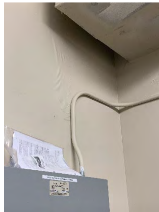
Figure 30 Building Headquarters First Floor (Room 108)
