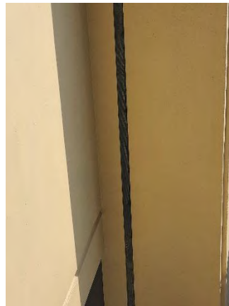
Figure 38 Bumby Ramp On
