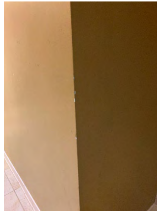
Figure 96 Building Headquarters First Floor (R.R. 100)
