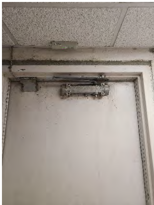
Figure 41 University Ramp Off
