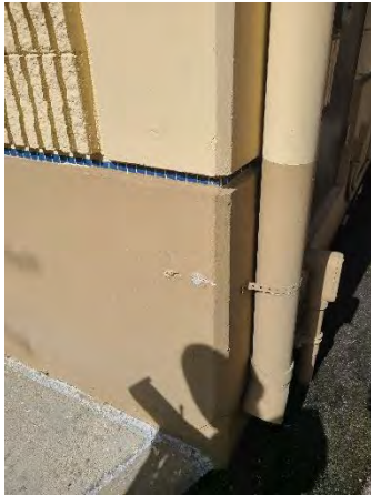
Figure 61 Mills Ramp Off
