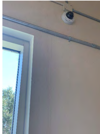
Figure 80 Building Headquarters First Floor (Stair 157)
