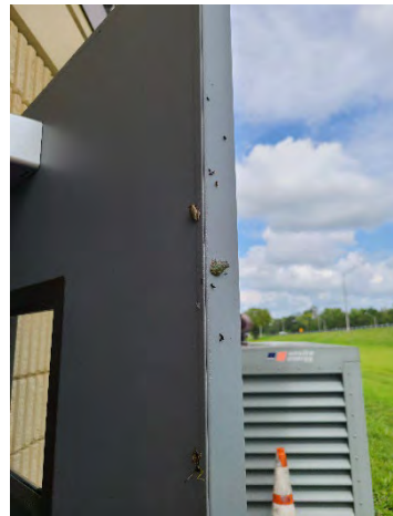
Figure 54 Dallas Ramp Off
