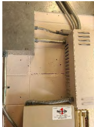
Figure 54 OB T Ramp Off
