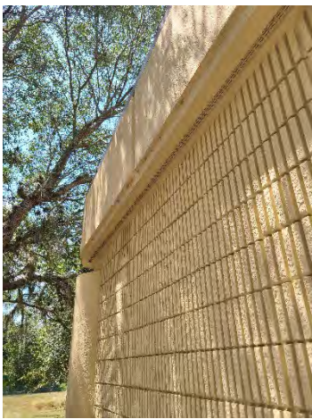
Figure 17 Forest Lake Mainline
