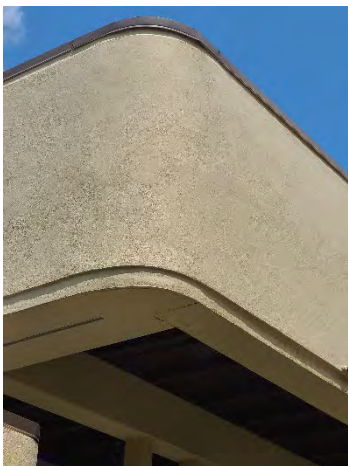
Figure 29 Forest Lake Mainline
