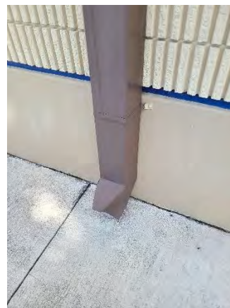
Figure 48 Conway Ramp On
