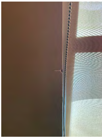
Figure 27 Building Headquarters First Floor (Room 107)
