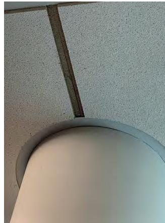
Figure 132 Building Headquarters Second Floor (Room 239)
