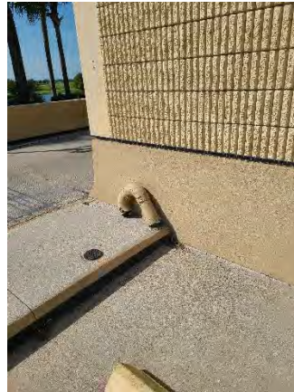
Figure 38 Lake Nona Ramp On
