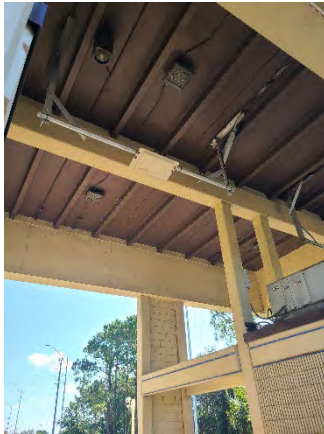
Figure 27 John Young Pkwy Ramp-On
