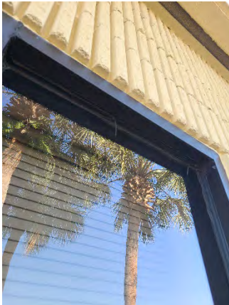
Figure 13 John Young Pkwy Mainline
