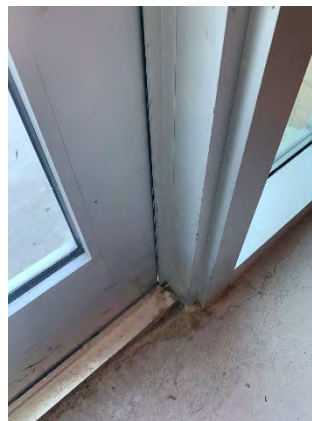
Figure 42 Building Headquarters First Floor (Room 132)
