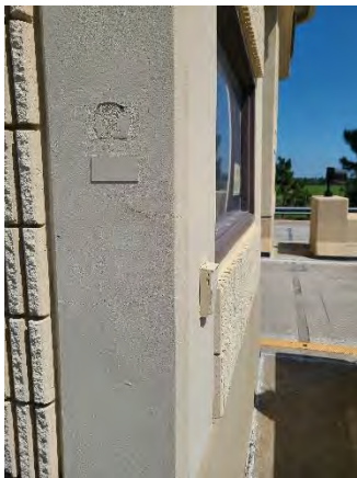
Figure 29 South Access Ramp Off
