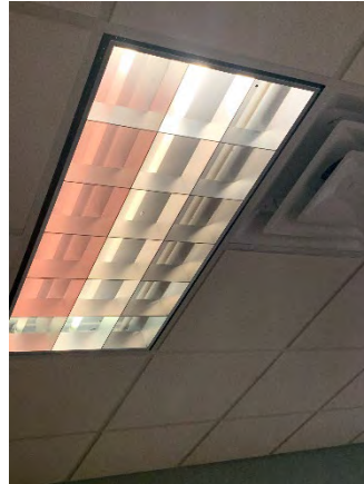
Figure 128 Building Headquarters Second Floor (Room 238)
