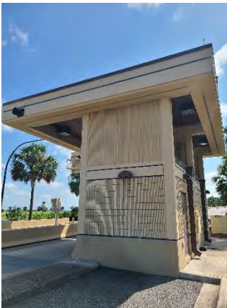
Figure 47 Conway Ramp On
