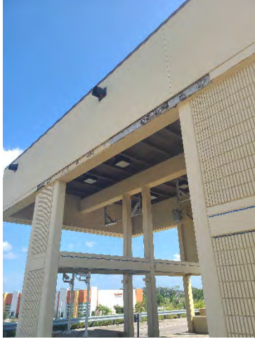
Figure 37 SR-438 Ramp Off
