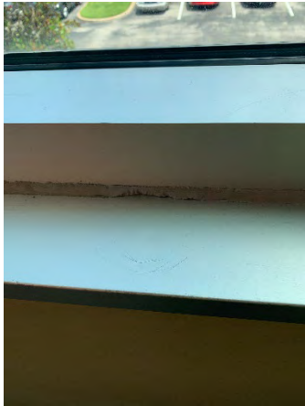
Figure 139 Building Headquarters Second Floor (Stair 248)
