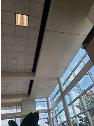
Figure 211 Building Headquarters Third Floor (Lobby 302)
