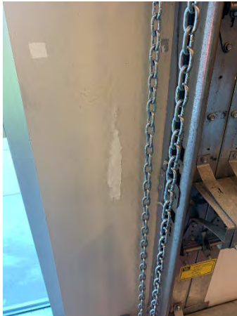
Figure 43 Building Headquarters First Floor (Room 132)
