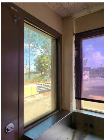
Figure 35 SR-438 Ramp On
