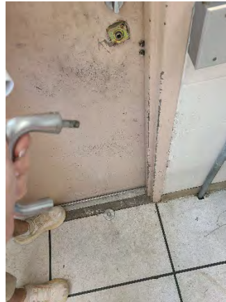
Figure 20 John Young Pkwy Ramp-Off
