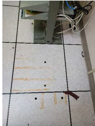
Figure 2 John Young Pkwy Mainline
