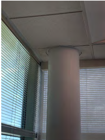
Figure 133 Building Headquarters Second Floor (Room 241)
