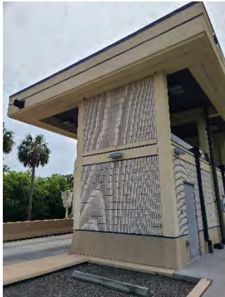
Figure 43 Conway Ramp Off
