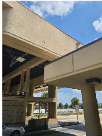
Figure 26 Forest Lake Mainline
