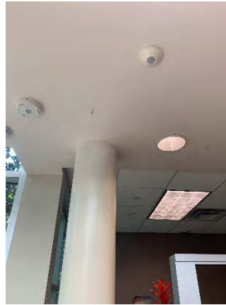
Figure 94 Building Headquarters First Floor (Lobby 117)
