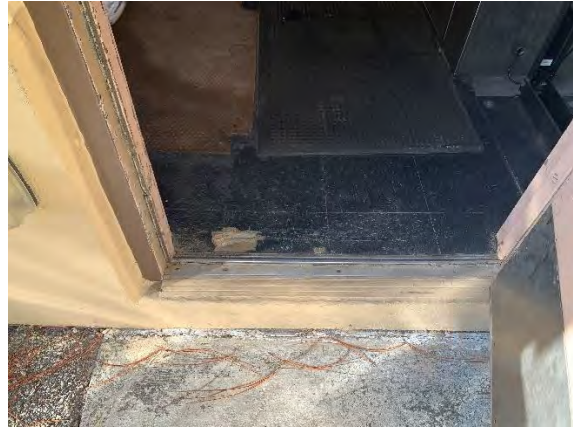
Figure 50 Hiawassee Ramp On
