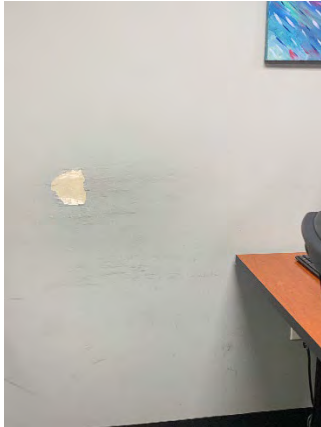
Figure 115 Building Headquarters Second Floor (Room 230)
