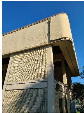
Figure 24 Lee Vista Ramp On
