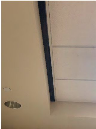
Figure 51 Building Headquarters First Floor (Room 136)
