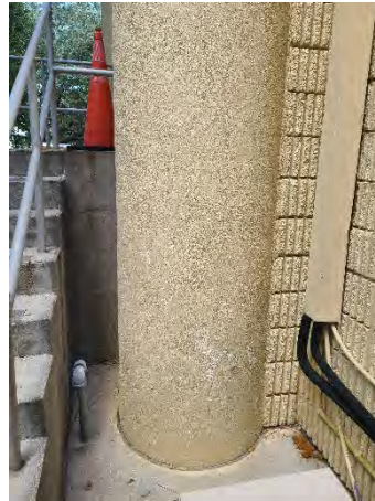
Figure 20 Forest Lake Mainline
