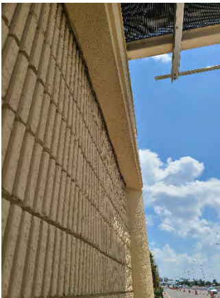
Figure 11 Forest Lake Mainline
