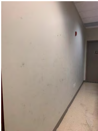
Figure 39 Building Headquarters First Floor (Room 129)
