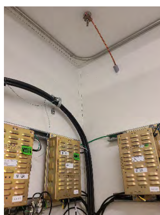
Figure 6 Marigold AET Toll Plaza
