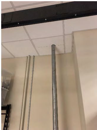
Figure 63 Building Headquarters First Floor (Room 144)
