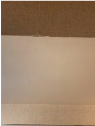
Figure 97 Building Headquarters First Floor (R.R. 100)
