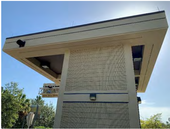
Figure 39 Good Homes Ramp Off
