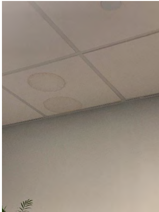
Figure 121 Building Headquarters Second Floor (Room 233)
