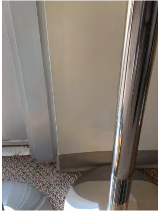
Figure 67 Building Headquarters First Floor (Room 150)
