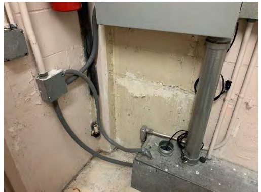
Figure 48 Hiawassee Ramp Off
