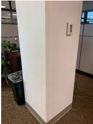
Figure 55 Building Headquarters First Floor (Room 142)
