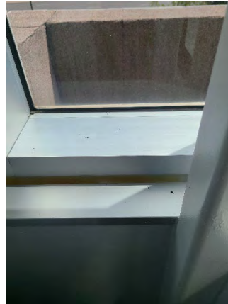
Figure 194 Building Headquarters Third Floor (Room 352B)
