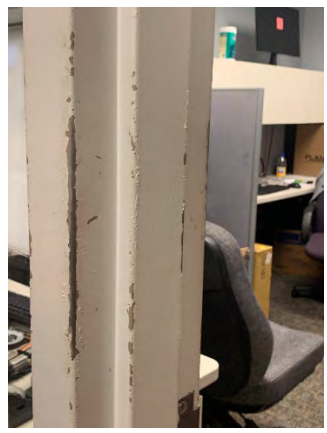
Figure 112 Building Headquarters Second Floor (Room 228)
