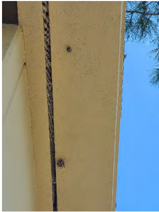
Figure 37 University Ramp Off
