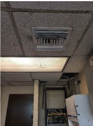
Figure 23 Boggy Creek Ramp On
