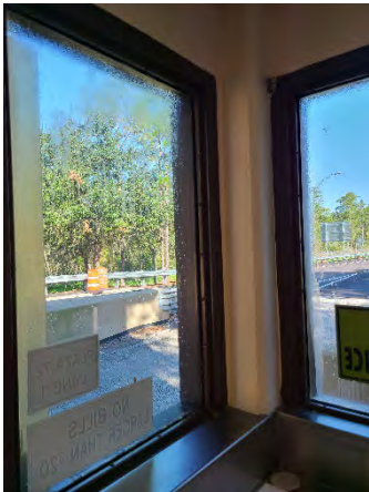
Figure 27 Lee Vista Ramp On
