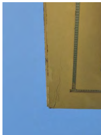
Figure 42 John Young Parkway Ramp Off
