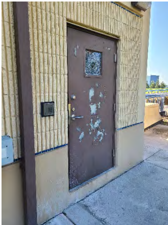
Figure 33 Lee Vista Ramp Off
