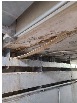
Figure 18 Lee Vista Ramp On
