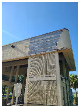
Figure 30 Lee Vista Ramp Off
