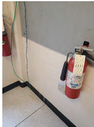
Figure 52 CR-437A Ramp Off
