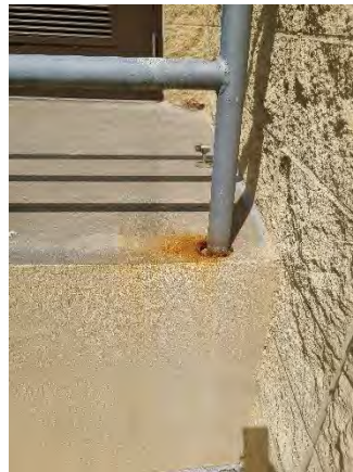
Figure 26 Conway EB Mainline
