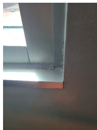
Figure 192 Building Headquarters Third Floor (Room 352B)
