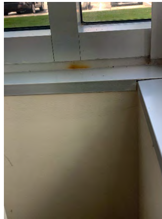
Figure 82 Building Headquarters First Floor (Stair 157)
