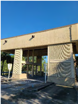
Figure 23 Lee Vista Ramp On
