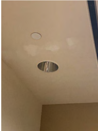
Figure 49 Building Headquarters First Floor (Room 136)
