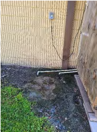
Figure 15 Boggy Creek Mainline
