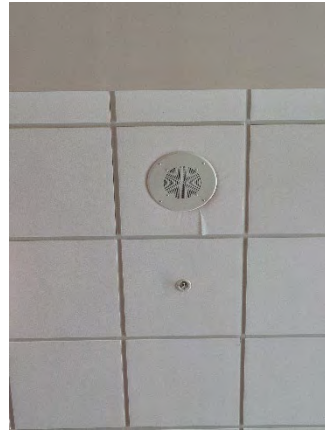
Figure 214 Building Headquarters Third Floor (Lobby 302)
