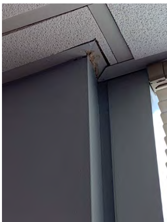
Figure 137 Building Headquarters Second Floor (Room 246)
