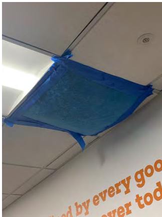
Figure 143 Building Headquarters Second Floor (Room 252)
