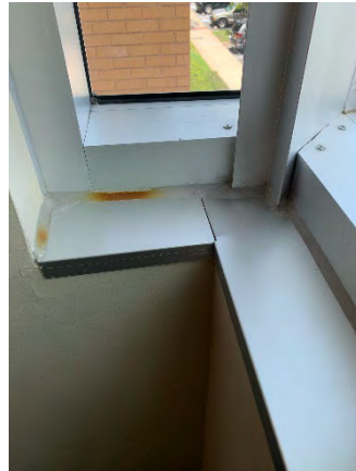
Figure 140 Building Headquarters Second Floor (Stair 248)
