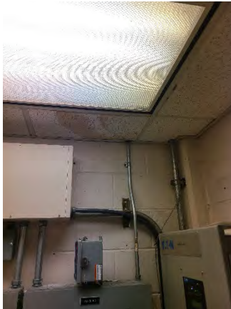
Figure 25 John Young Pkwy Ramp-On
