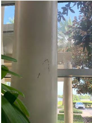
Figure 93 Building Headquarters First Floor (Lobby 117)
