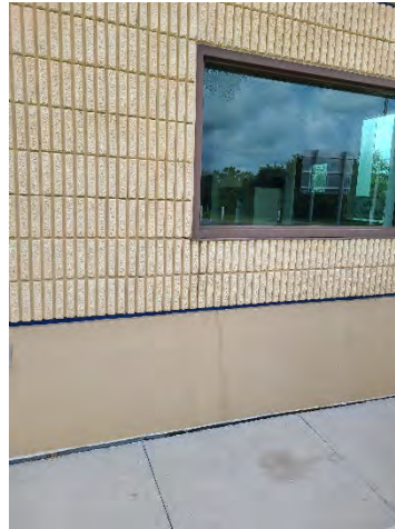
Figure 52 Dallas Ramp Off
