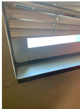
Figure 84 Building Headquarters First Floor (Room 160)
