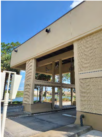
Figure 31 SR-438 Ramp On
