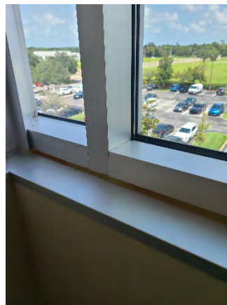
Figure 210 Building Headquarters Third Floor (Stair 358)
