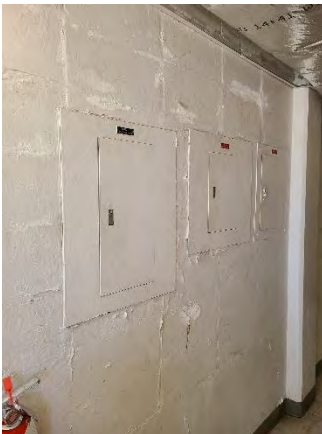
Figure 35 Dean Ramp On
