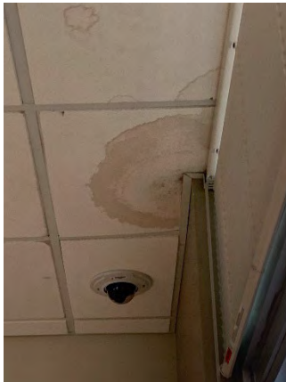
Figure 45 Building Headquarters First Floor (Room 135)
