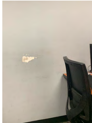
Figure 116 Building Headquarters Second Floor (Room 230)
