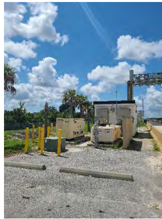
Figure 10 KOA AET Toll Plaza
