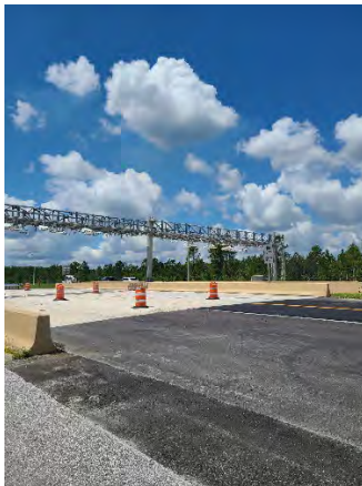
Figure 9 KOA AET Toll Plaza
