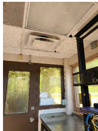
Figure 42 University Ramp Off
