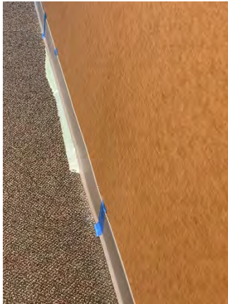
Figure 145 Building Headquarters Second Floor (Corr. 256)
