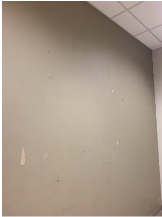
Figure 31 Building Headquarters First Floor (Room 119)
