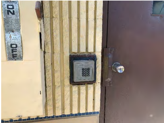
Figure 49 Hiawassee Ramp On
