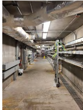
Figure 14 Conway EB Mainline
