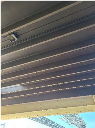
Figure 15 John Young Pkwy Mainline
