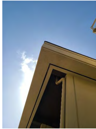
Figure 62 Mills Ramp Off
