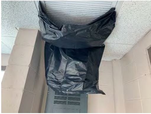
Figure 43 Good Homes Ramp Off
