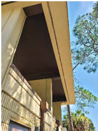
Figure 35 University Ramp Off
