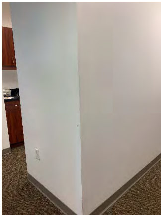
Figure 59 Building Headquarters First Floor (Room 142)
