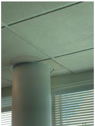
Figure 131 Building Headquarters Second Floor (Room 239)
