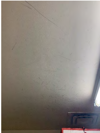
Figure 25 Building Headquarters First Floor (Room 104)
