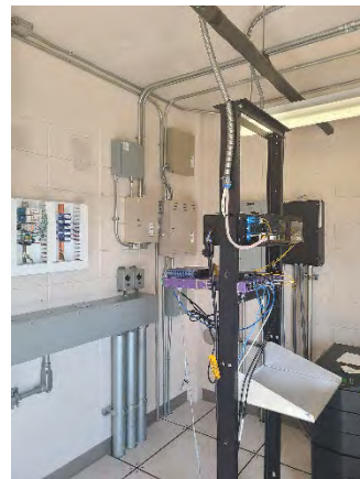
Figure 42 SR-438 Ramp Off
