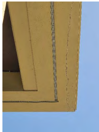
Figure 40 John Young Parkway Ramp Off
