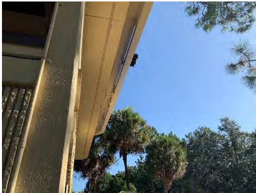
Figure 45 Hiawassee Ramp Off
