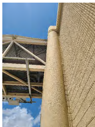
Figure 12 Forest Lake Mainline
