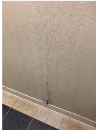
Figure 148 Building Headquarters Second Floor (R.R. 201)
