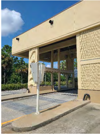
Figure 43 West Road Ramp On
