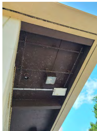
Figure 36 University Ramp Off
