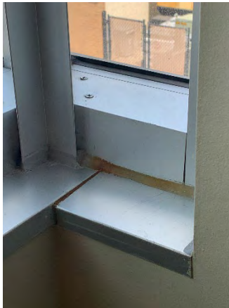
Figure 123 Building Headquarters Second Floor (Stair 234)
