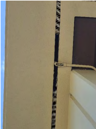
Figure 49 OB T Ramp Off
