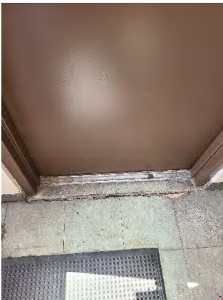
Figure 51 OB T Ramp Off
