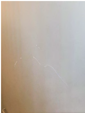
Figure 141 Building Headquarters Second Floor (Stair 248)
