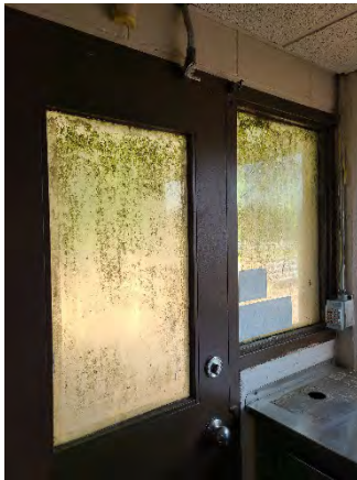
Figure 39 University Ramp Off
