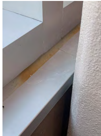
Figure 78 Building Headquarters First Floor (Room 156)
