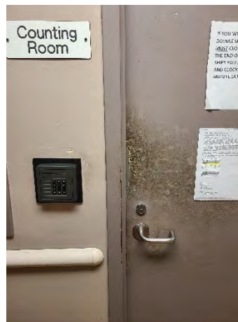
Figure 6 Forest Lake Mainline
