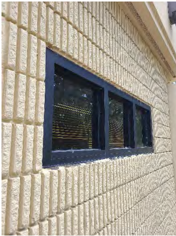
Figure 21 Forest Lake Mainline
