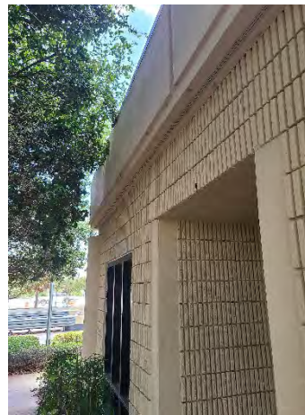
Figure 18 Forest Lake Mainline
