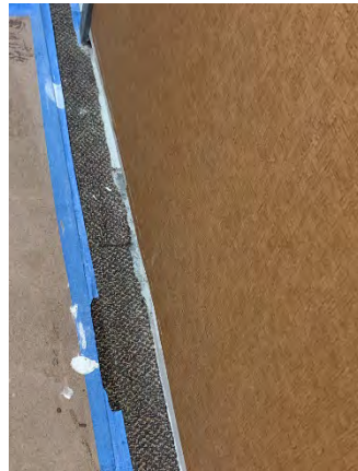
Figure 144 Building Headquarters Second Floor (Corr. 256)
