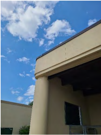
Figure 21 Conway EB Mainline
