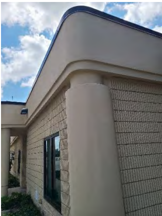
Figure 23 Conway EB Mainline
