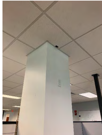
Figure 56 Building Headquarters First Floor (Room 142)
