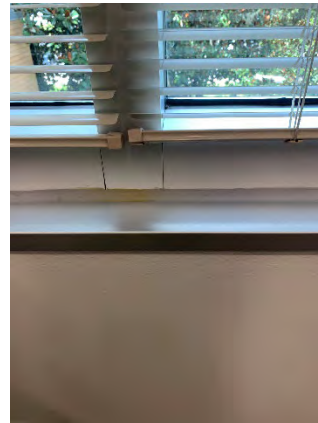
Figure 106 Building Headquarters Second Floor (Room 219)
