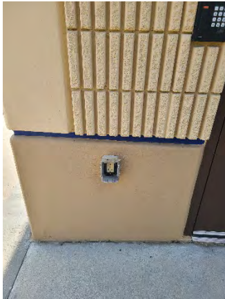
Figure 49 CR-437A Ramp Off
