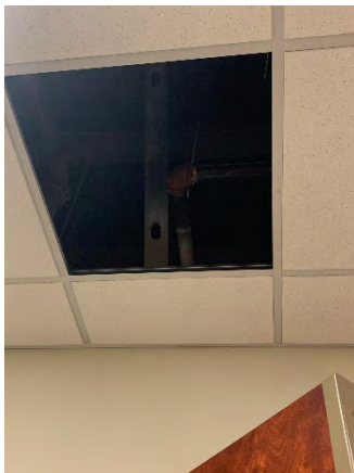
Figure 35 Building Headquarters First Floor (Room 127)
