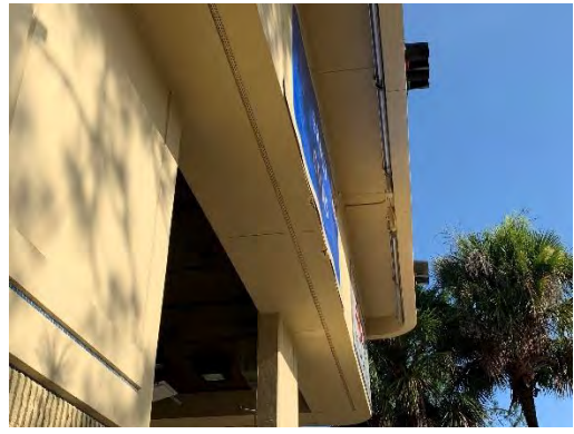
Figure 46 Hiawassee Ramp Off
