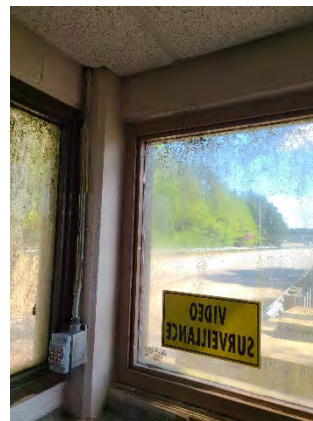
Figure 40 University Ramp Off
