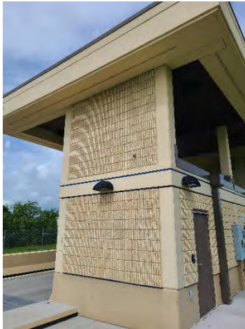
Figure 49 Dallas Ramp Off
