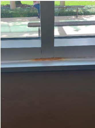
Figure 75 Building Headquarters First Floor (Room 156)
