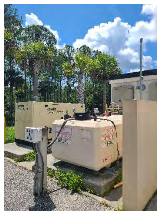
Figure 4 Marigold AET Toll Plaza
