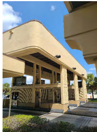
Figure 28 Forest Lake Mainline
