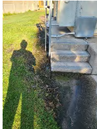
Figure 14 Boggy Creek Mainline
