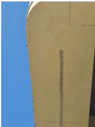
Figure 41 SR-438 Ramp Off
