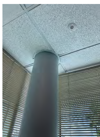
Figure 126 Building Headquarters Second Floor (Room 235)
