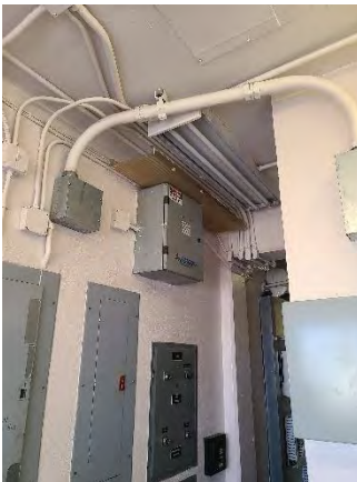
Figure 53 Conway Ramp Off
