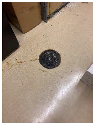
Figure 64 Building Headquarters First Floor (Room 149)
