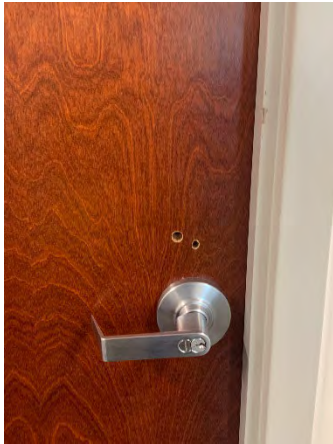
Figure 127 Building Headquarters Second Floor (Room 237)
