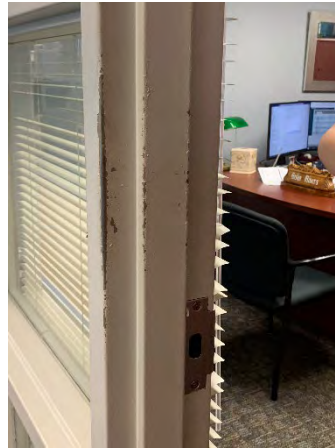
Figure 134 Building Headquarters Second Floor (Room 242)
