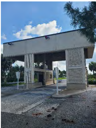
Figure 21 John Young Pkwy Ramp-Off
