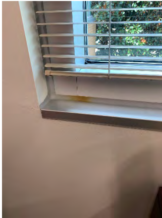
Figure 105 Building Headquarters Second Floor (Room 219)
