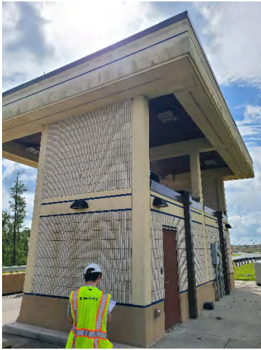
Figure 61 ICP Ramp Off
