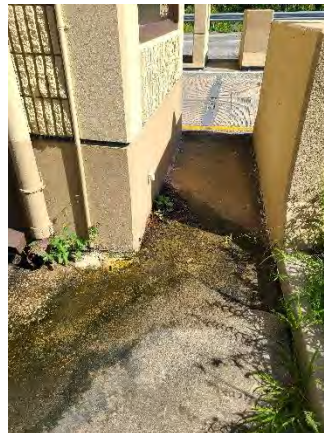
Figure 32 Dean Ramp On
