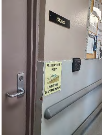
Figure 1 Boggy Creek Mainline
