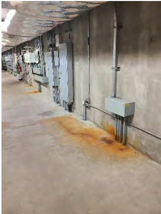
Figure 23 Conway EB Mainline
