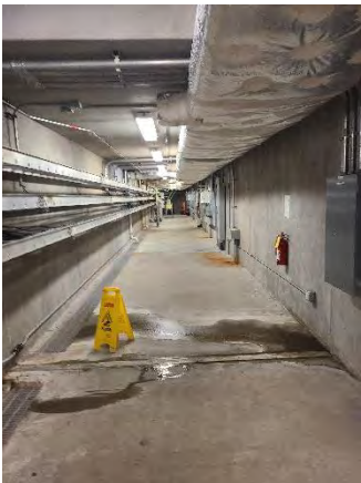
Figure 11 Conway EB Mainline
