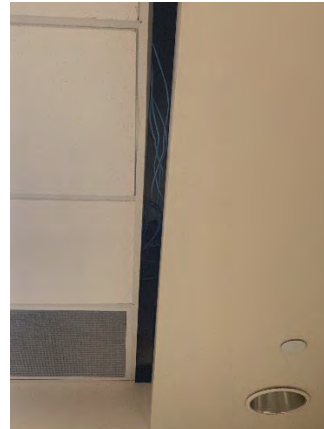
Figure 50 Building Headquarters First Floor (Room 136)
