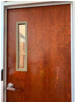
Figure 107 Building Headquarters Second Floor (Room 219)
