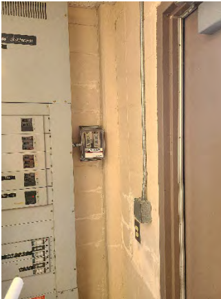
Figure 63 CR-535 Ramp On
