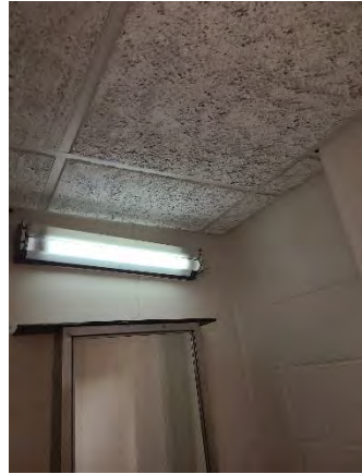
Figure 64 Mills Ramp Off
