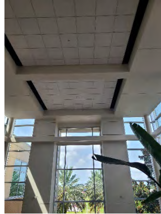
Figure 212 Building Headquarters Third Floor (Lobby 302)
