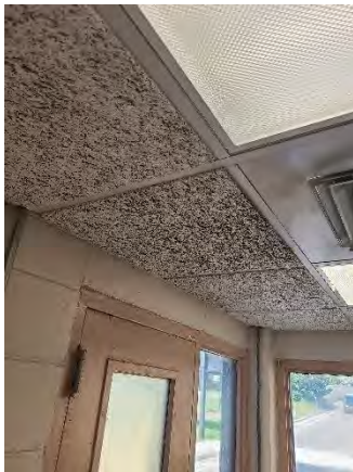
Figure 65 Mills Ramp Off
