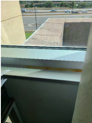
Figure 195 Building Headquarters Third Floor (Room 352B)
