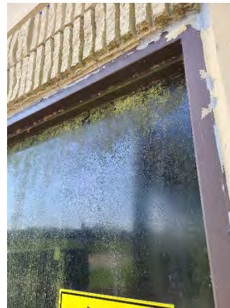
Figure 38 University Ramp Off
