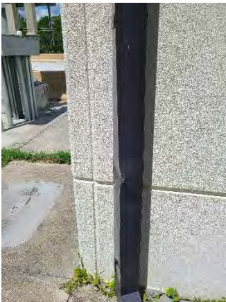
Figure 5 Marigold AET Toll Plaza
