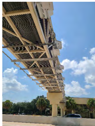
Figure 10 Forest Lake Mainline
