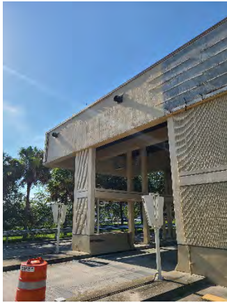
Figure 31 Lee Vista Ramp Off
