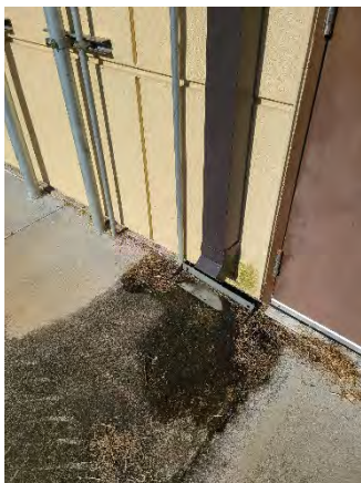
Figure 59 Mt. Ponkan Gantry
