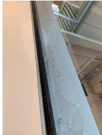
Figure 110 Building Headquarters Second Floor (Room 222)
