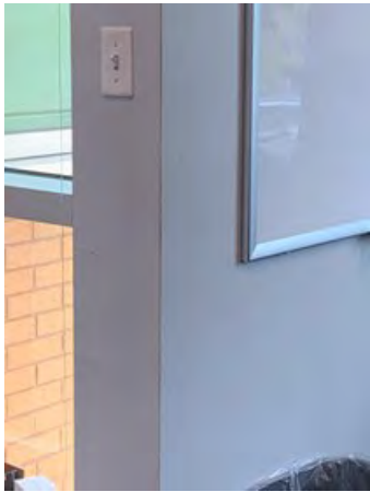
Figure 135 Building Headquarters Second Floor (Room 243)
