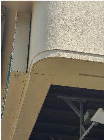
Figure 25 Forest Lake Mainline
