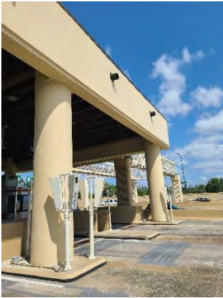
Figure 27 Conway EB Mainline
