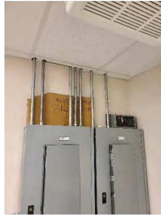
Figure 2 Conway EB Mainline
