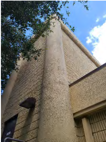
Figure 39 Forest Lake Mainline
