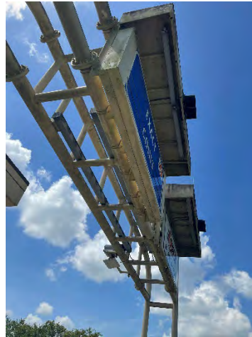
Figure 50 Dallas Ramp Off
