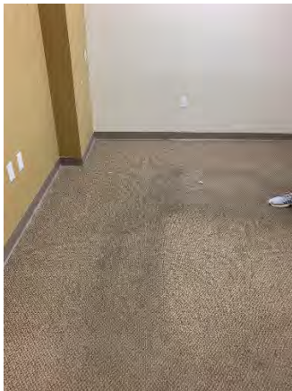
Figure 33 Building Headquarters First Floor (Room 120)
