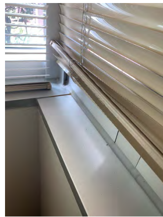
Figure 52 Building Headquarters First Floor (Room 137)
