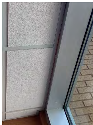
Figure 124 Building Headquarters Second Floor (Stair 234)
