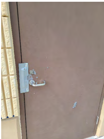
Figure 53 Dallas Ramp Off
