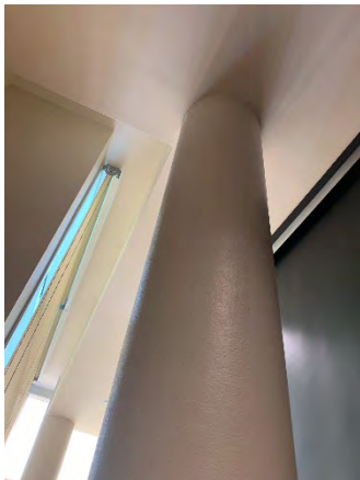
Figure 29 Building Headquarters First Floor (Room 107)
