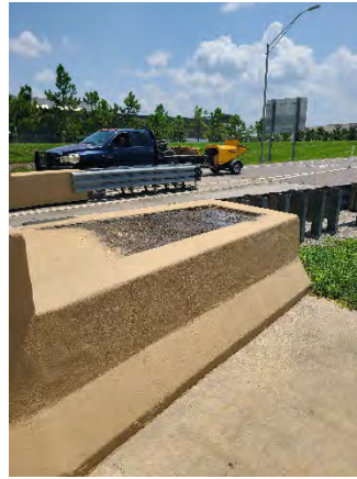
Figure 50 New Independence Ramp Off
