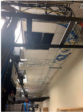
Figure 62 Building Headquarters First Floor (Room 144)
