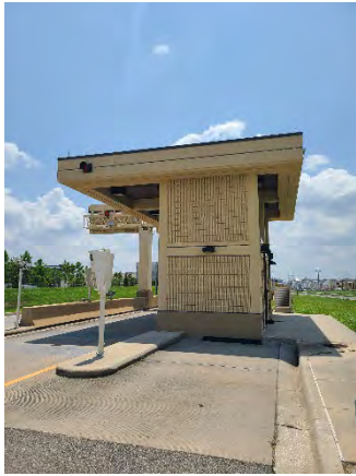
Figure 49 New Independence Ramp Off
