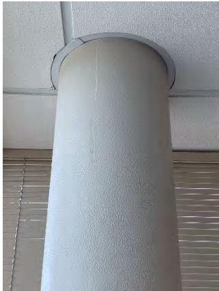
Figure 117 Building Headquarters Second Floor (Room 231)
