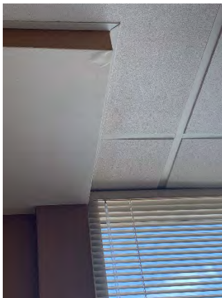
Figure 119 Building Headquarters Second Floor (Room 231)
