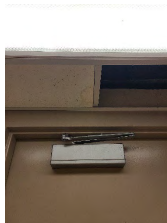
Figure 40 Schofield Ramp On
