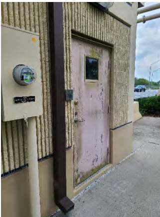
Figure 59 CR-535 Ramp On
