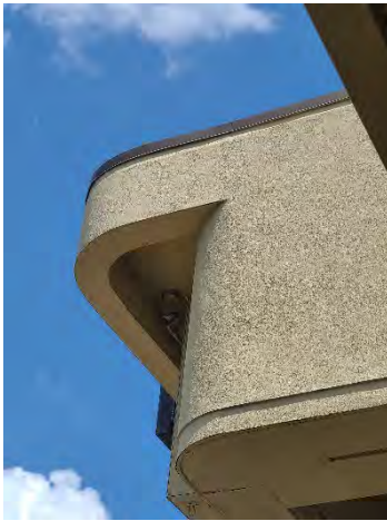
Figure 27 Forest Lake Mainline
