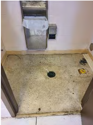
Figure 49 Conway Ramp On
