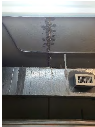
Figure 9 Boggy Creek Mainline
