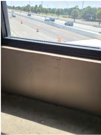
Figure 15 Forest Lake Mainline
