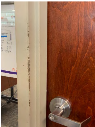
Figure 113 Building Headquarters Second Floor (Room 230)
