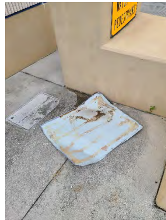
Figure 38 Schofield Ramp On
