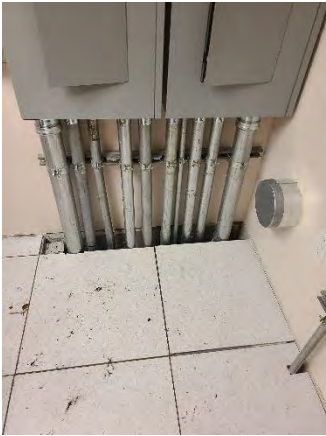
Figure 3 Conway EB Mainline
