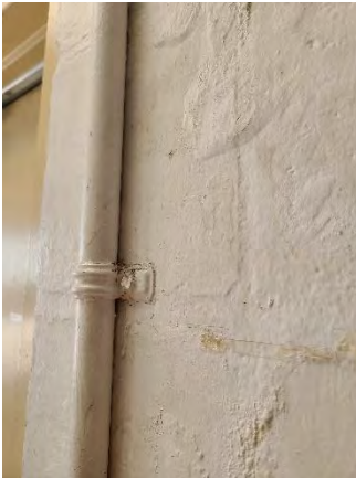
Figure 33 Dean Ramp On
