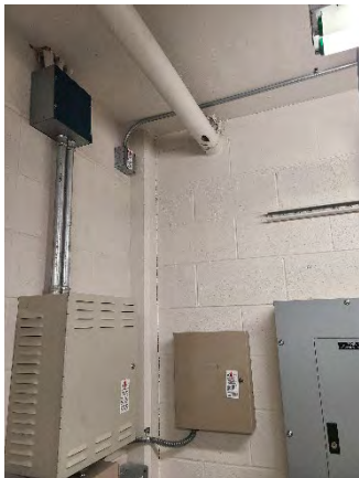
Figure 29 Lee Vista Ramp On
