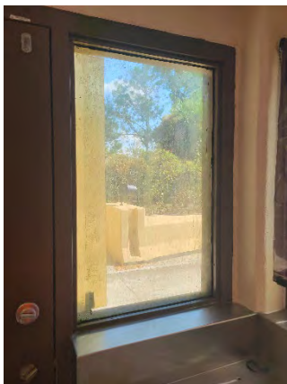
Figure 47 West Road Ramp Off
