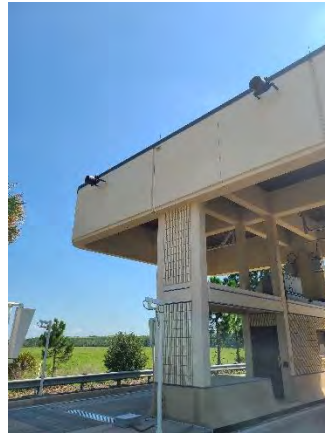
Figure 26 South Access Ramp Off
