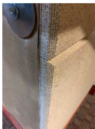
Figure 72 Building Headquarters First Floor (Room 156)
