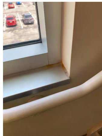
Figure 138 Building Headquarters Second Floor (Stair 248)
