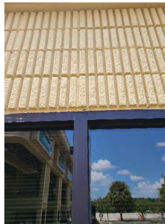
Figure 24 Forest Lake Mainline
