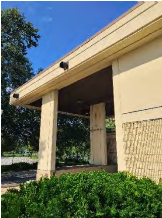
Figure 51 Conway Ramp Off
