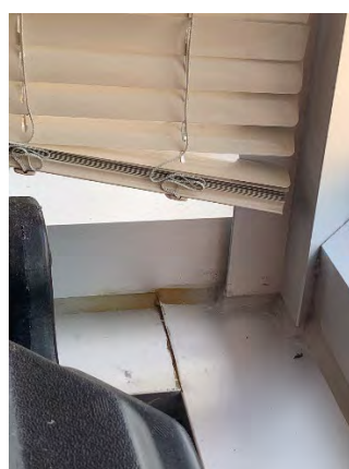
Figure 120 Building Headquarters Second Floor (Room 231)
