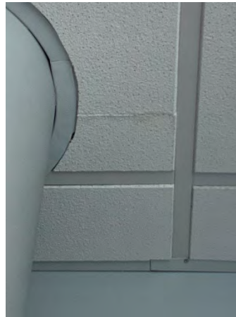
Figure 136 Building Headquarters Second Floor (Room 246)
