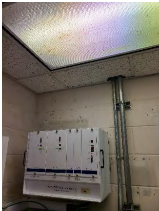
Figure 23 John Young Pkwy Ramp-On
