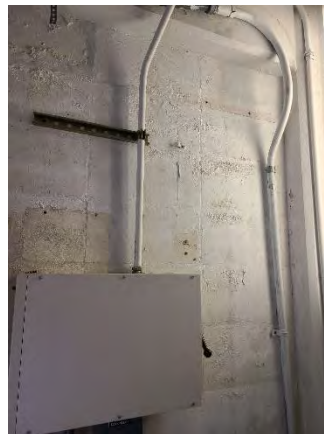
Figure 36 Dean Ramp On
