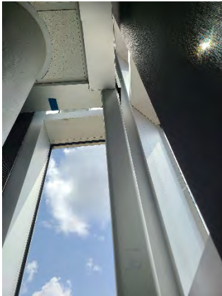
Figure 193 Building Headquarters Third Floor (Room 352B)
