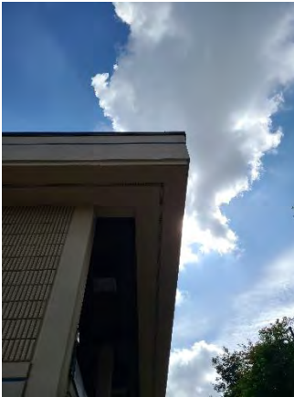
Figure 39 Hiwassee Ramp Off
