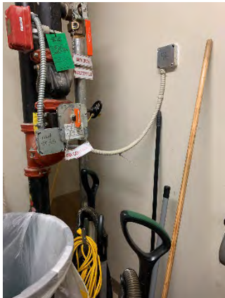
Figure 101 Building Headquarters Second Floor (Room 205)
