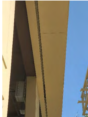
Figure 50 OB T Ramp Off
