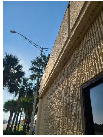
Figure 12 Boggy Creek Mainline
