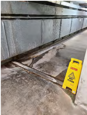
Figure 17 Lee Vista Ramp On
