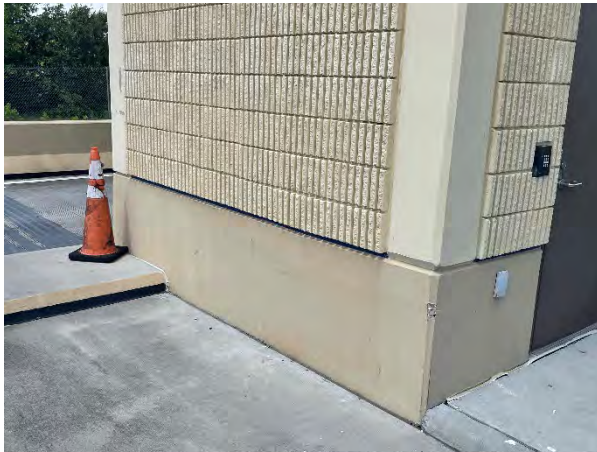
Figure 51 Dallas Ramp Off
