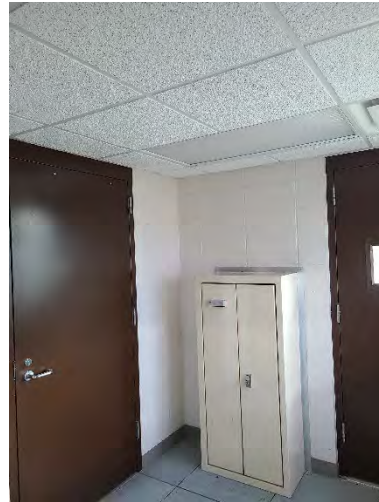
Figure 64 ICP Ramp Off
