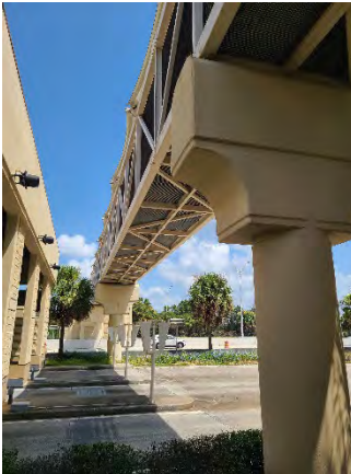
Figure 9 Forest Lake Mainline
