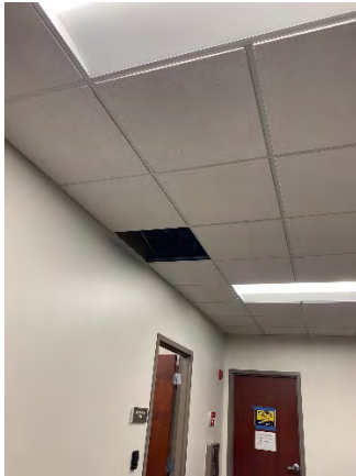
Figure 111 Building Headquarters Second Floor (Room 222)
