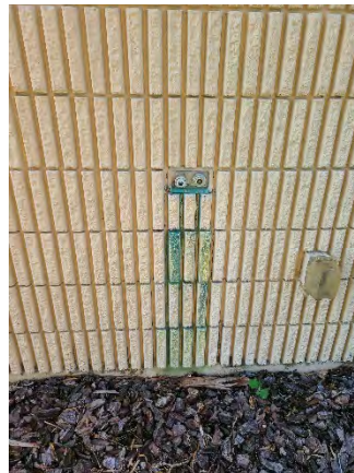
Figure 14 John Young Pkwy Mainline
