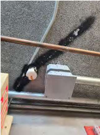
Figure John Young Pkwy Mainline
