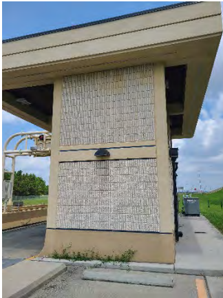
Figure 37 Schofield Ramp On
