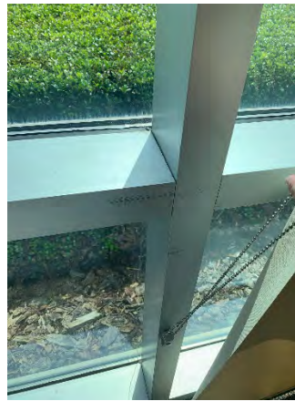
Figure 28 Building Headquarters First Floor (Room 107)
