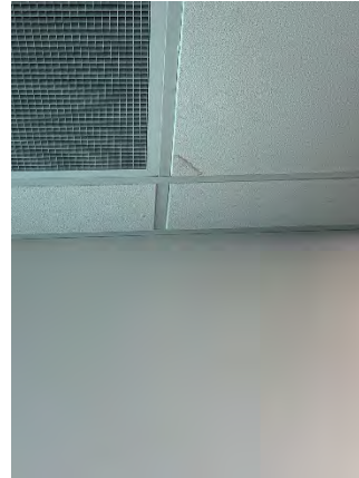
Figure 104 Building Headquarters Second Floor (Room 219)
