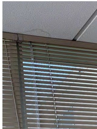
Figure 118 Building Headquarters Second Floor (Room 231)
