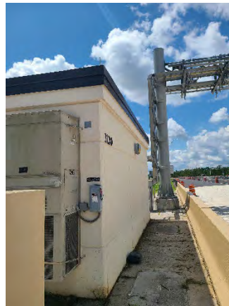
Figure 2 Marigold AET Toll Plaza
