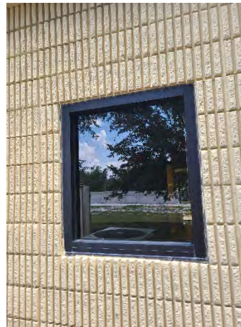
Figure 22 Forest Lake Mainline
