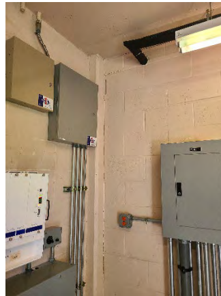
Figure 66 CR-535 Ramp On
