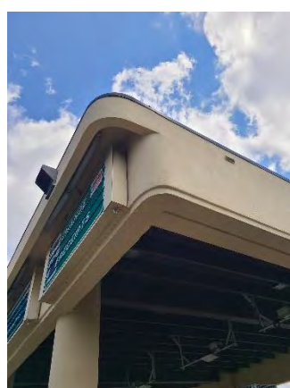
Figure 24 Conway EB Mainline
