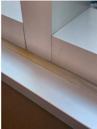
Figure 79 Building Headquarters First Floor (Room 156)
