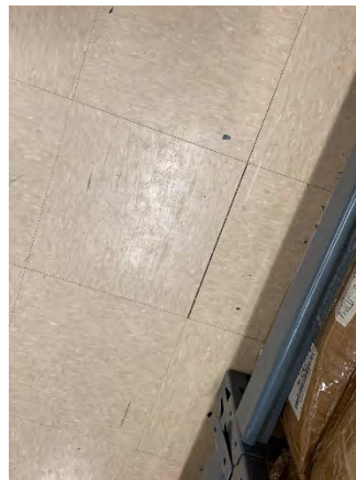
Figure 36 Building Headquarters First Floor (Room 127)
