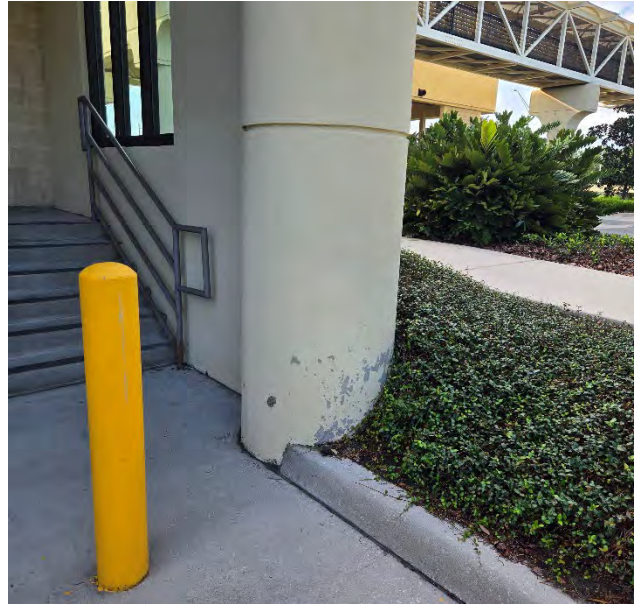
FIGURE 8: Damaged coatings Coral Hills Mainline Plaza
