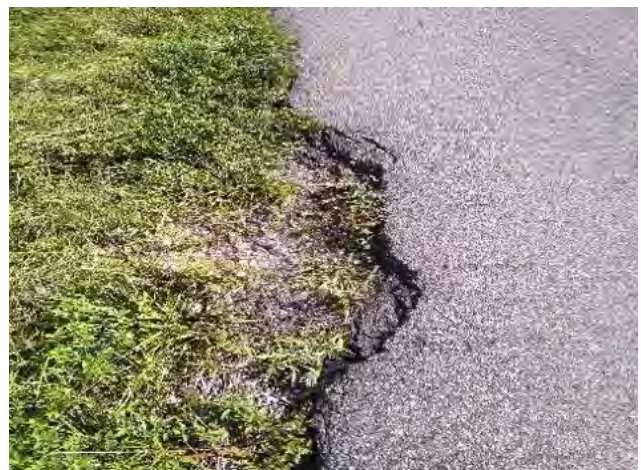
FIGURE 9: Pavement edge ravel SR 408 and SR 417 Interchange
