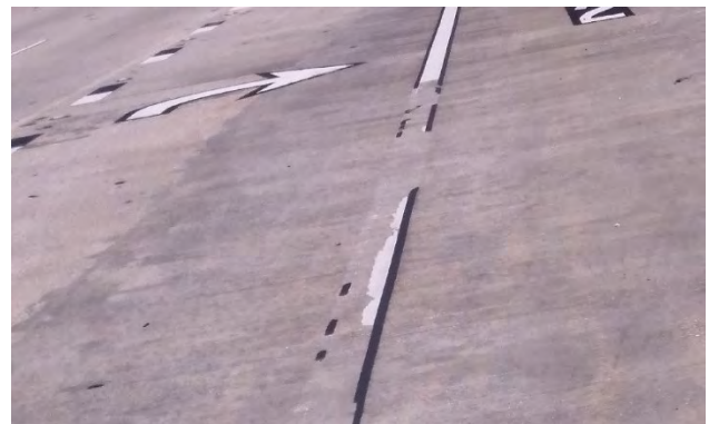
FIGURE 4: Pavement marking deterioration bridge over Lake Sherwood
