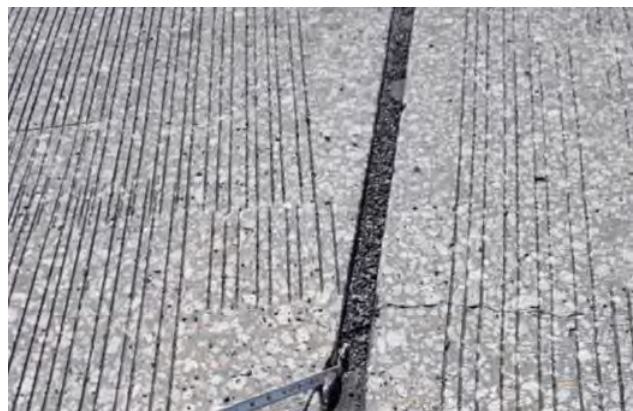
FIGURE 7: Adhesion loss at abutment joint bridge over CR437A
