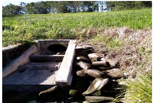
FIGURE 6: Erosion around drainage structure in pond at Keene Road
