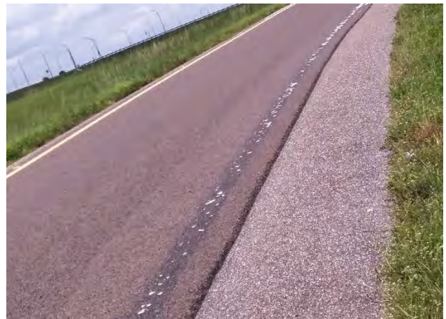
FIGURE 12: Lane striping degradation Schofield Road on ramp
