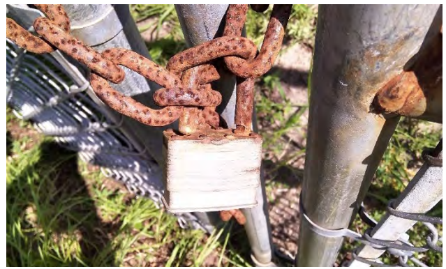
FIGURE 14: Inoperable gate lock SR 451
