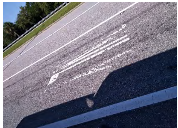
FIGURE 16: Pavement degradation SR 551 Goldenrod Road north of SR 528
