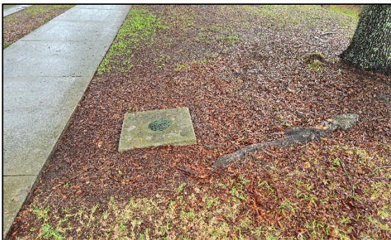
Photo 2.9. Example of buried water line utility along Red Cleveland Boulevard, facing northwest.
