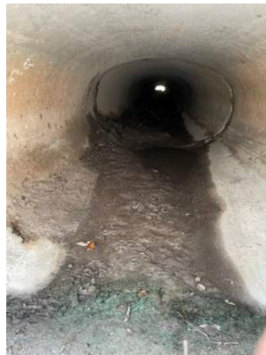
Photo 16: View inside of elliptical pipe of CD-04_EX looking south. Some sedimentation and stain lines were observed.
