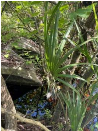
Photo 21: View of south (downstream) mitered endwall (ST-13) of CD-06_EX. Endwall was observed to be in good condition and had no apparent scour or erosion. The water level for ST-13 was approximately 6-inches above the pipe invert. The structure had no sedimentation (silt), nor any observed stain lines.
