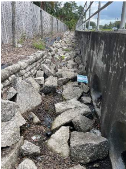
Photo 15: View of ditch with stone revetment upstream CD-04_EX looking east.
