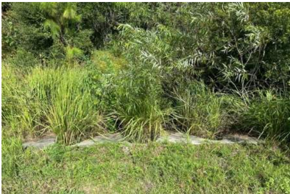
Photo 19: View of southeast (downstream) mitered endwall (ST-11) of CD-05_EX. Endwall was observed to be in good condition and had no apparent scour or erosion. The structure had vegetation, there was no sedimentation (silt), and no stain lines were observed.
