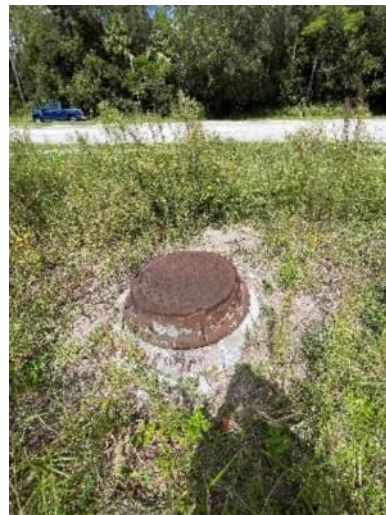
Photo 12: View of storm manhole (ST-6) which joins CD_03A and CD_03B at the downstream side. From manhole, a 38" x 60" ERCP conveys runoff within Sylvestri Lakes Community and outfalls into a wetland area located east of the community.
