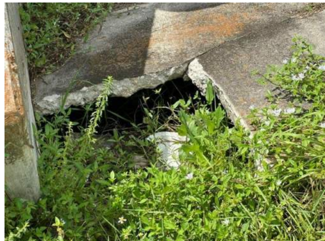
Photo 8: View of scour on the headwall structure of triple 48-inch pipes. This structure is located at East Lake Mary Blvd approximately 100-ft west of Mellonville Avenue.
