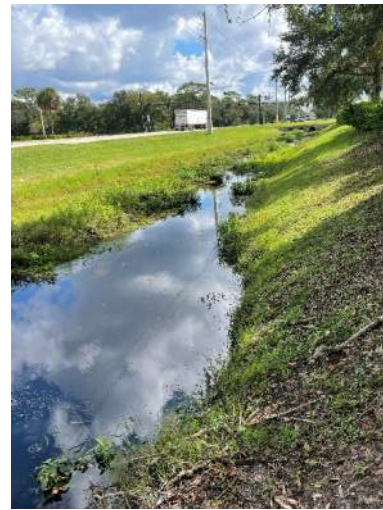
Photo 6: View east of roadside ditch downstream of triple 48-inch side drain which conveys the runoff from CD-02_EX and other areas to triple 48-inch pipes.
