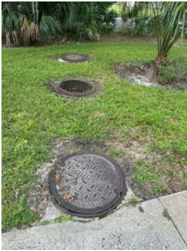
Photo 9: View of manholes structures corresponding to a triple 48-inch pipes which conveys the runoff from the roadside ditch to a downstream wetland. These structures are located at Mellonville Avenue approximately 640-ft south of East Lake Mary Blvd, on the west side next to the sidewalk just before the beginning of a tall concrete wall.
