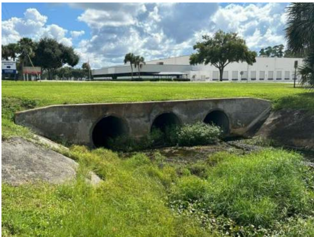
Photo 7: View southeast of triple 48-inch pipes which receive the runoff from the roadside ditch and conveys the runoff to a downstream wetland. This structure is located at East Lake Mary Blvd approximately 100-ft west of Mellonville Avenue.
