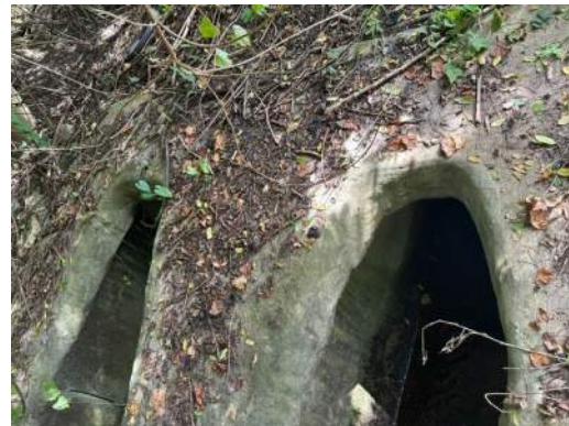
Photo 20: View of north (upstream) mitered endwall (ST-12) of CD-06_EX. Endwall was observed to be in good condition and had no apparent scour or erosion. The water level for ST-12 was approximately 6-inches above the pipe invert. The structure had no sedimentation (silt), nor any observed stain lines.
