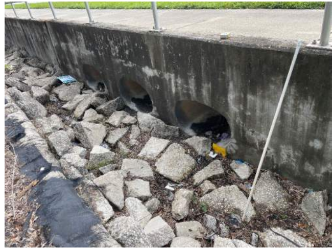
Photo 14: View of north (upstream) endwall (ST-8) of CD-04_EX. Endwall was observed to be in good condition and had no apparent scour or erosion. There was no standing water or flow on the day of the field review. The structure had no sedimentation (silt), nor any observed stain lines.
