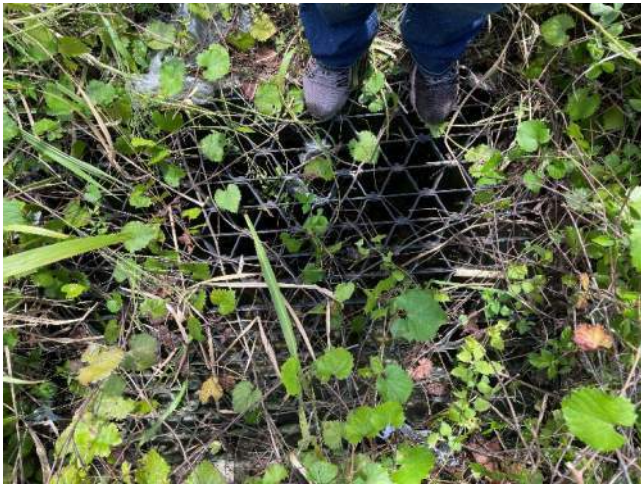
Photo 13: View of north (upstream) ditch bottom inlet (ST-7) of CD-03B_EX. Ditch bottom inlet was observed to be in good condition and had no apparent scour or erosion. There was no standing water or flow on the day of the field review.
