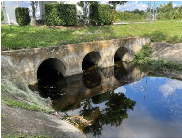
Photo 5: View northwest of triple 48-inch side drain downstream of CD-02_EX which conveys the runoff to an roadside ditch.
