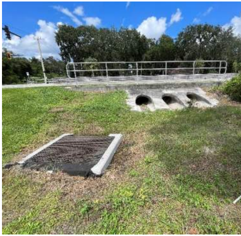
Photo 17: View of south (downstream) endwall (ST-9) of CD-04_EX. Endwall was observed to be in good condition and had no apparent scour or erosion. There was no standing water or flow on the day of the field review. The structure had no sedimentation (silt), nor any observed stain lines. A DBI structure was observed downstream the endwall, however, it could not be determined in the field how it is related to the drainage system.
