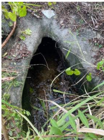
Photo 11: View of north (upstream) mitered endwall (ST-5) of CD-03A_EX. Endwall was observed to be in good condition and had no apparent scour or erosion. The water level and stain marks were measured at approximately 5-inches and 8-inches above the pipe invert, respectively.
