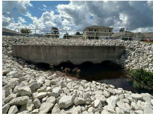
Photo 10: View of quadruple pipes structure which receive the runoff from the triple 48-inch pipes and conveys the runoff to a downstream wetland. This structure is located at Hidden Palm Dr. approximately 860-ft east of Mellonville Avenue.
